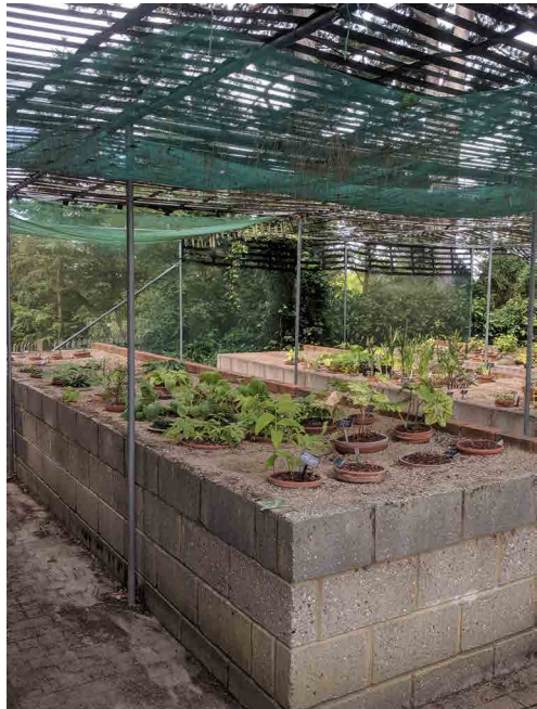
Durable plunge bed made from concrete blocks.
