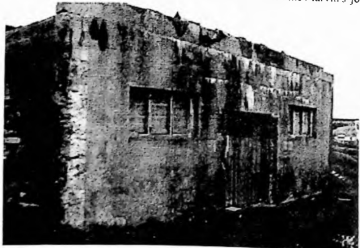
The forbidden entrance to the subterranean vault used for teaching techniques of using breathing apparatus whilst recovering casualties from smoke-filled darkened buildings.
