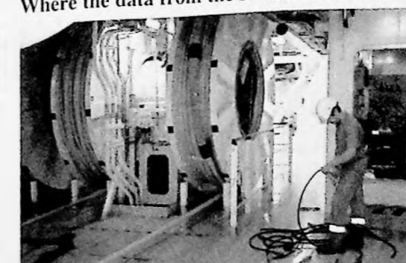
A worker dwarfed by the huge cable reels
