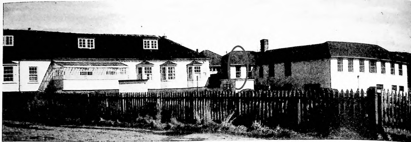
The original King Edward VII Memorial Hospital with additional solarium (left) and the Churchill Wing in the 1960s. Maternity ward window circled in red. Note chalets in the foreground Picture: Rowlands Collection
