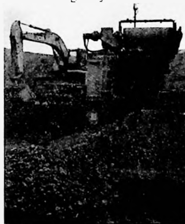
Crusher at work at the Port Harriet quarry
