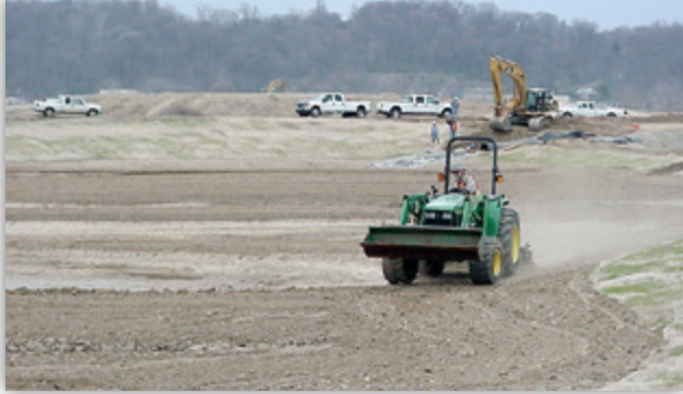
Site preparation for wetland mitigation, Cincinnati, OH
