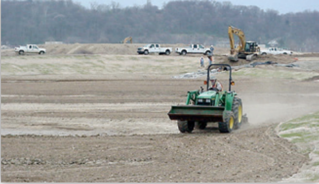
Site preparation for wetland mitigation, Cincinnati, OH
