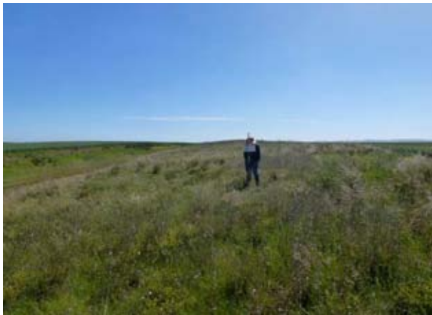
Photo 67: FRE-SHA-01, BS836, 21/10/12. Photo looking north. Rail cutting on left side.
