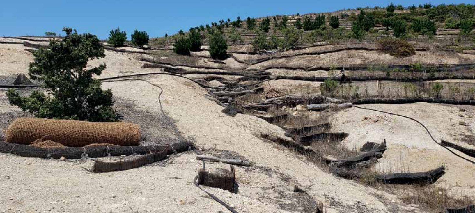
Check dams and wattles at the restoration site on Santa Rosa Island showing a healthy population of bishop pines.
