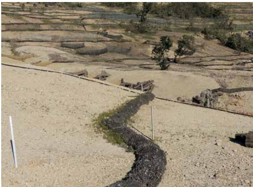
Wattles prevent erosion and support plant growth at the Santa Rosa Island restoration site.
