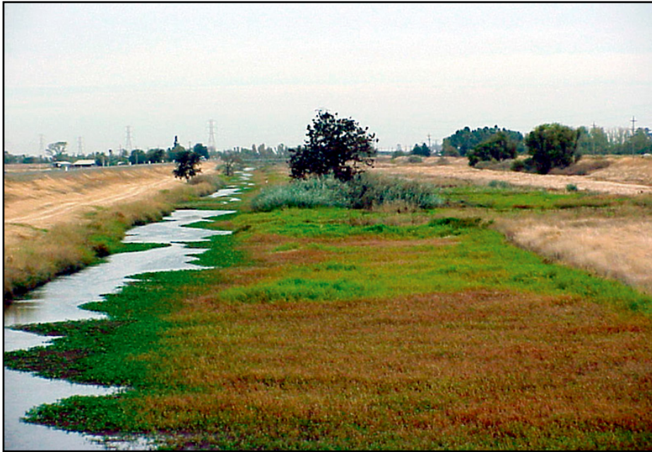
Steelhead Creek (formerly the Natomas East Main Drain Canal)
