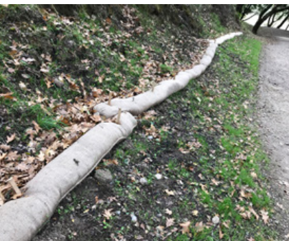
Straw wattles placed to slow and dissipate water, with rolls overlapping. Photo by Rich Casale
