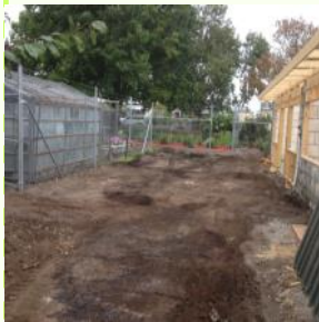
Nursery during construction in April 2013
