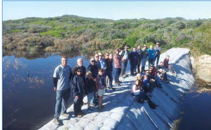
Figure 8.22 – NGT staff members celebrate the completion of the third and final sandbag structure with some of the many dedicated volunteers from the local community.
