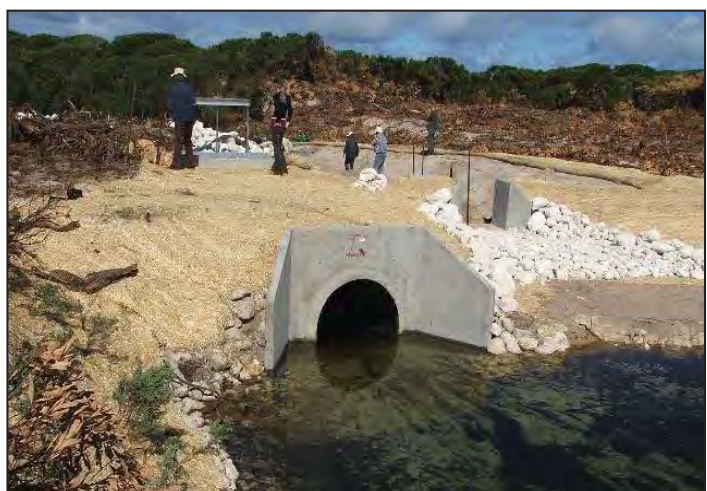
Figure 8.16 – Stage 1 weir and fishway under construction in 2006.
