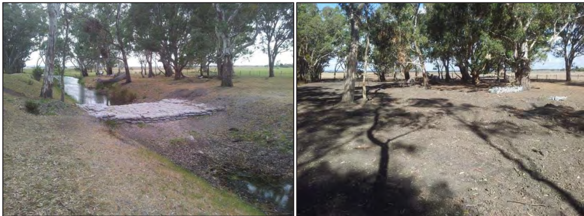
Figure 8.10 – Brady Swamp drain, trial structure before (left) & after (right) 2015 permanent works
