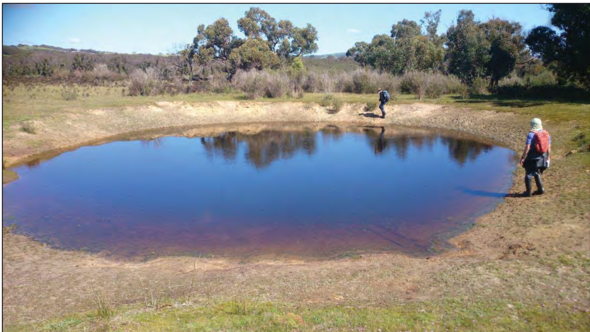
Figure 4.11 – The dam in Stipiturus CP, of 1980s construction, which intercepts hill-side seepage.
