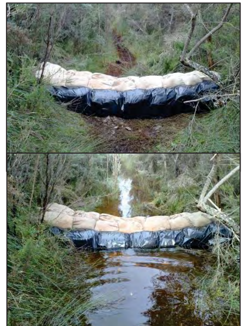
Figure 8.13 – an example of a block installed on the drain in Lake St Clair CP, before (above) and during (below) winter flows in 2009.
