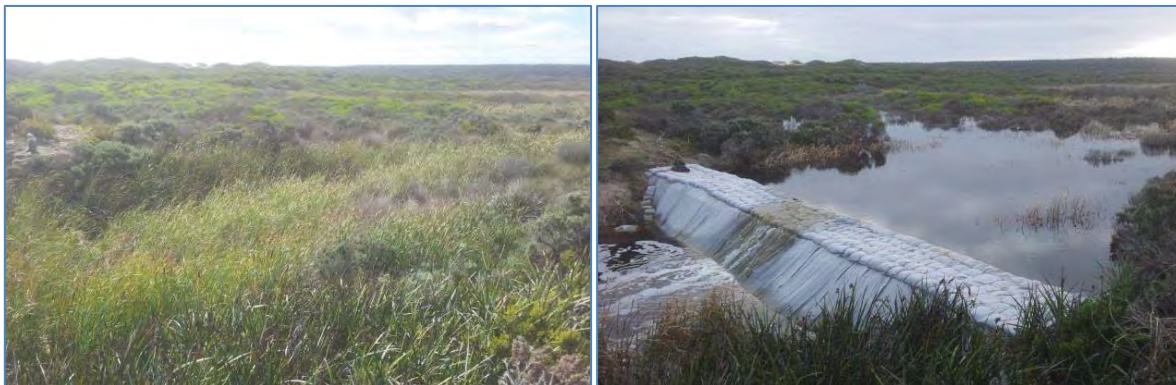
Figure 8.23 – View of the Phase 3 Restoration Trial Structure location; LEFT – prior to construction in March 2015, and RIGHT – in June 2015
