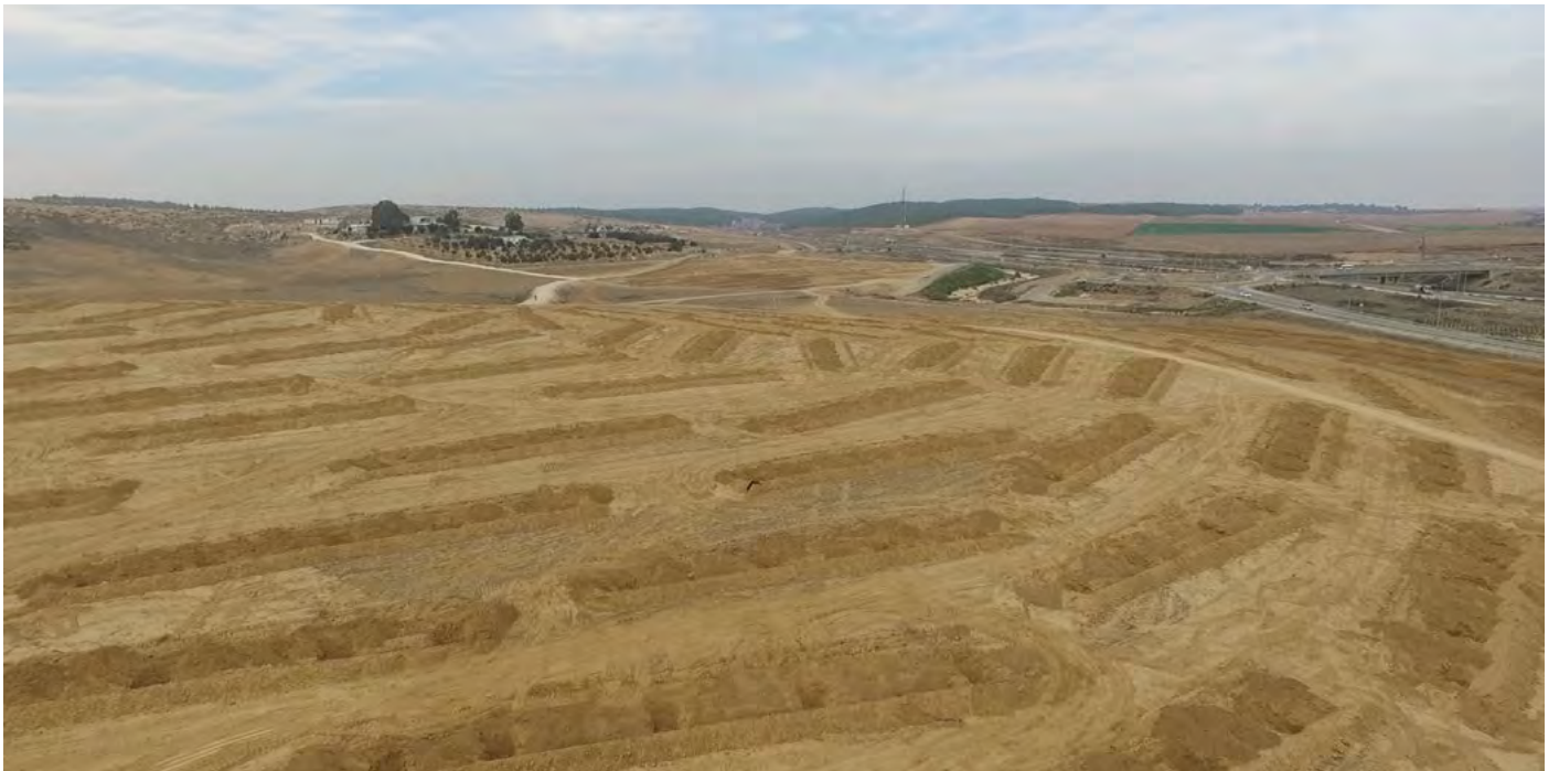
Pre-planting earthworks in a loess area in the Northern Negev. The natural vegetation and the soil crust have been completely removed. Photo: Yosef Segal
