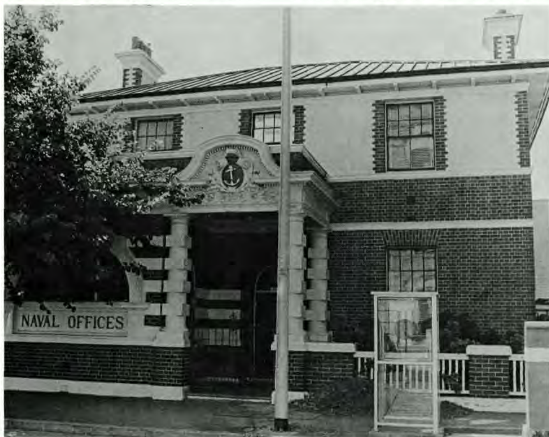
Naval Staff Office, Edward Street, Brisbane completed 1900 and vacated 1977. — by courtesy Defence Public Relations
