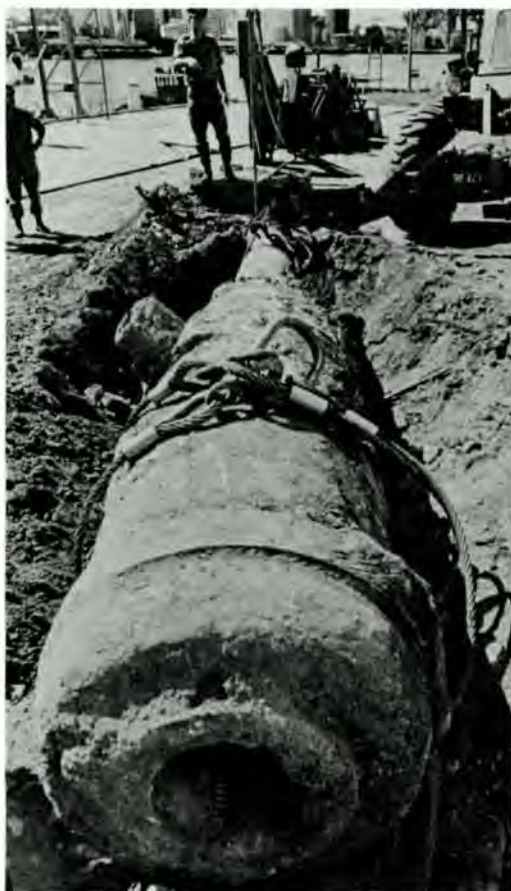
Excavation of one of GAYUNDAH 's 8" guns at Kangaroo Point — by courtesy Defence Public Relations
