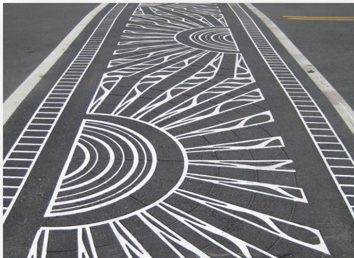
Crosswalk with epoxy resin
