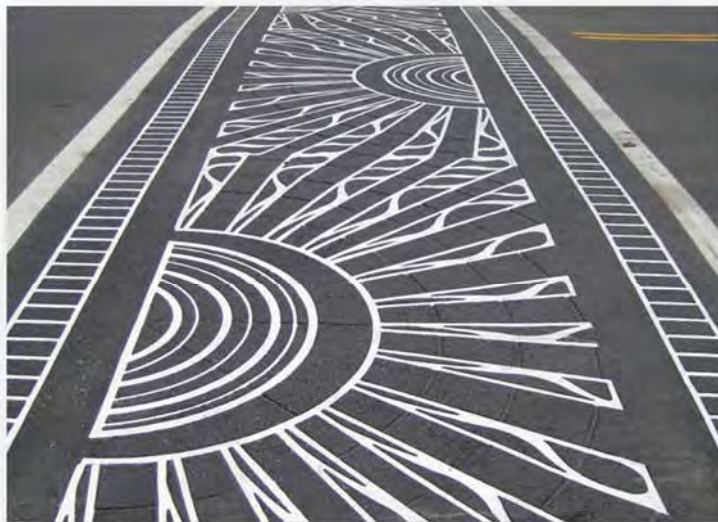
Crosswalk with epoxy resin
