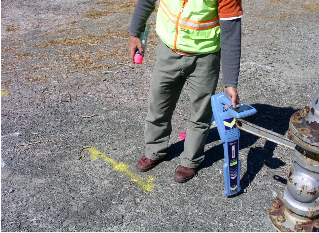
Photograph D-1. Utility locating and mark out
