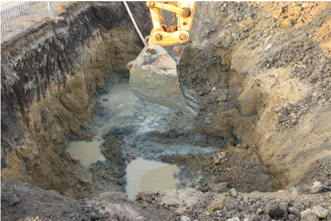
Photograph D-4. Excavating contaminated soil
