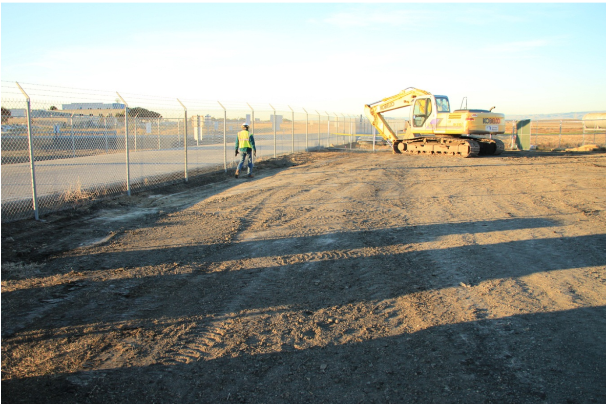
Photograph D-10. Final grade
