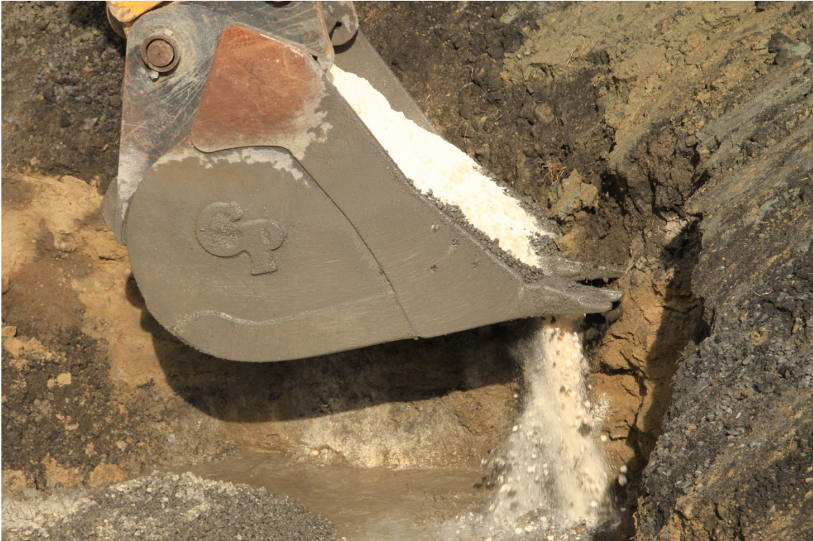
Photograph D-7. Adding ORC to crushed rock backfill
