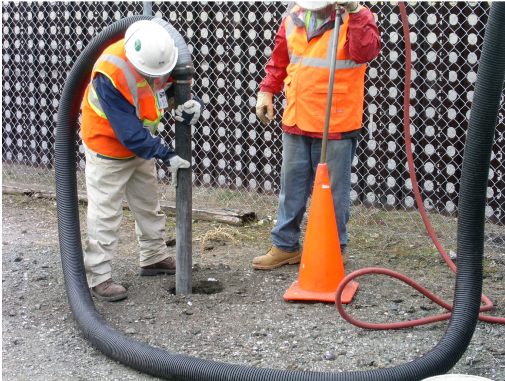
Photograph D-13. Vacuum excavation along Sump 63 pipeline
