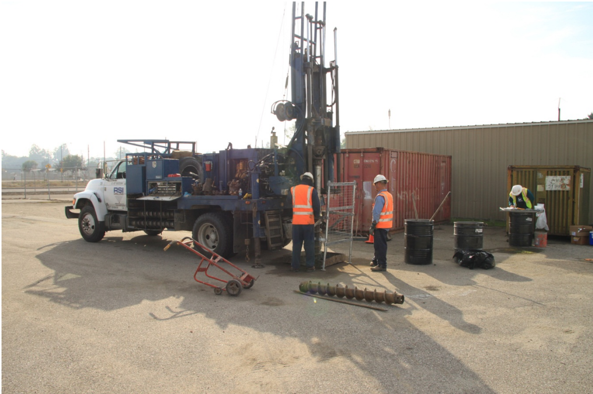
Photograph D-19. Well installation Former UST 58 (Bldg. 544 in background)
