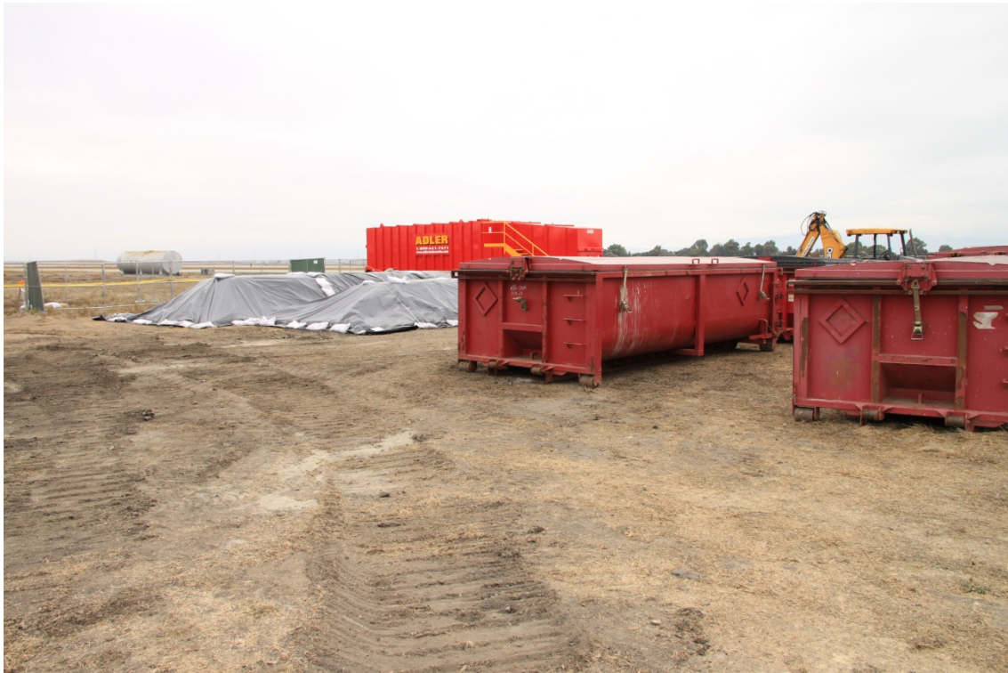
Photograph D-6. Clean overburden (covered), water tank, and roll-off bins
