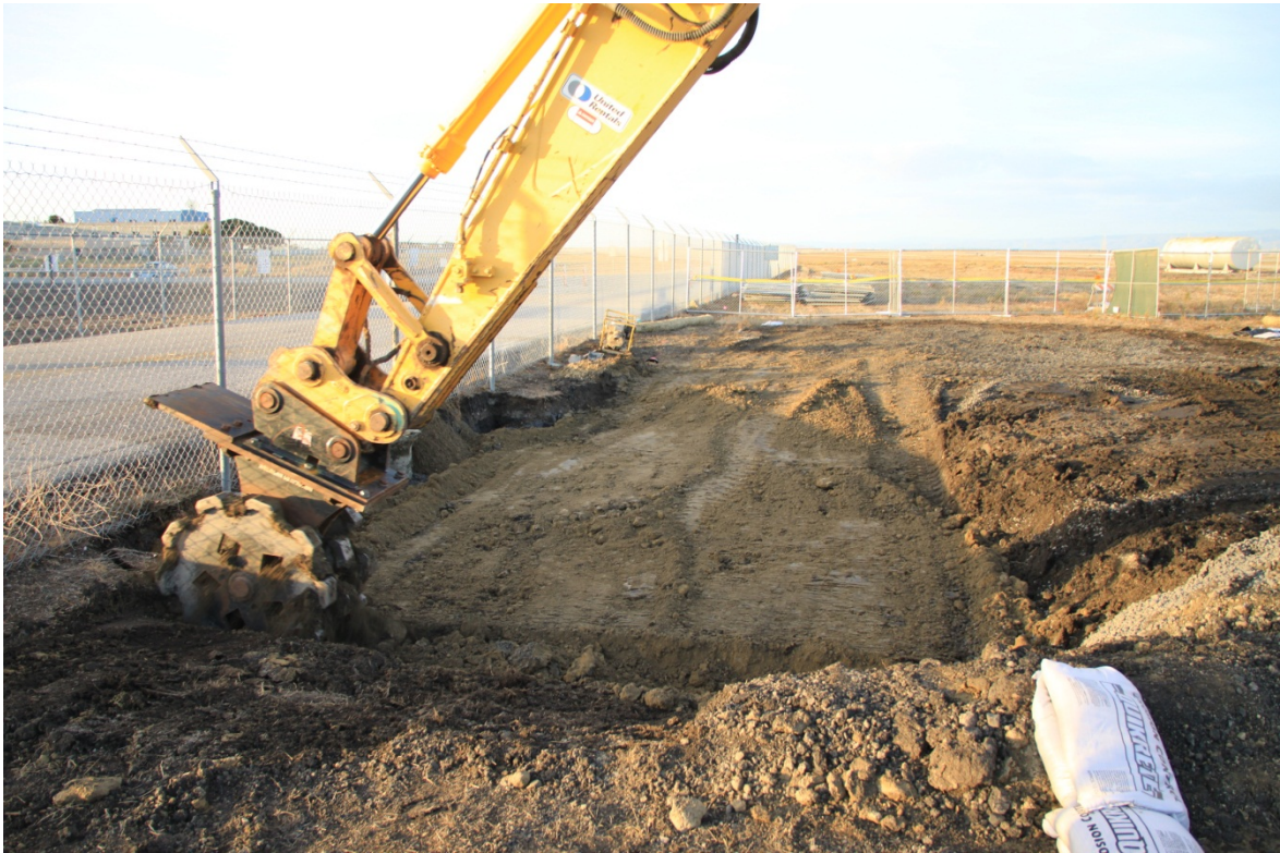
Photograph D-9. Compacting clean overburden
