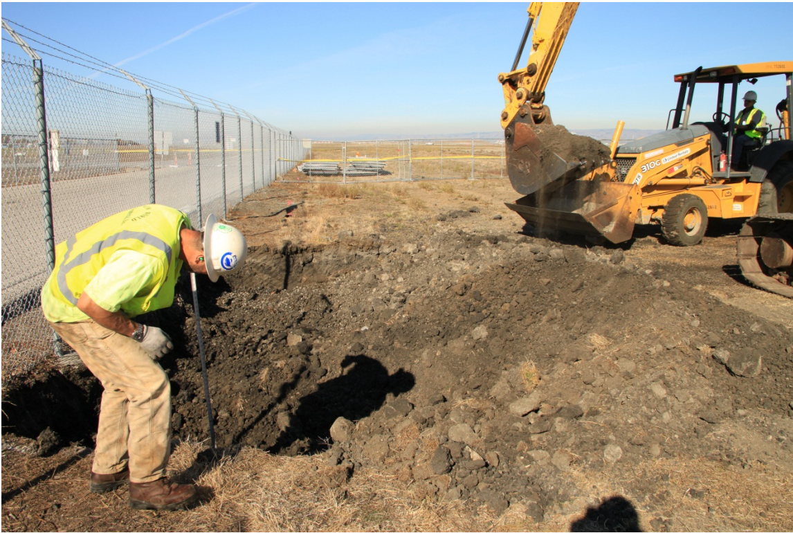
Photograph D-3. Removing and segregating clean overburden at Zook Rd
