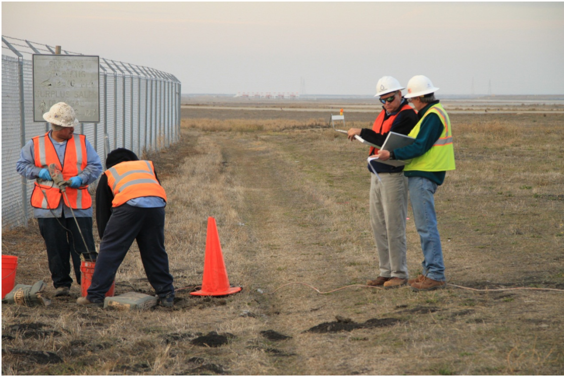
Photograph D-11. Santa Clara Water District Inspector visit during well installation
