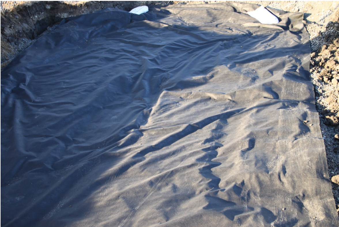
Photograph D-8. Geotextile fabric on top of crushed rock
