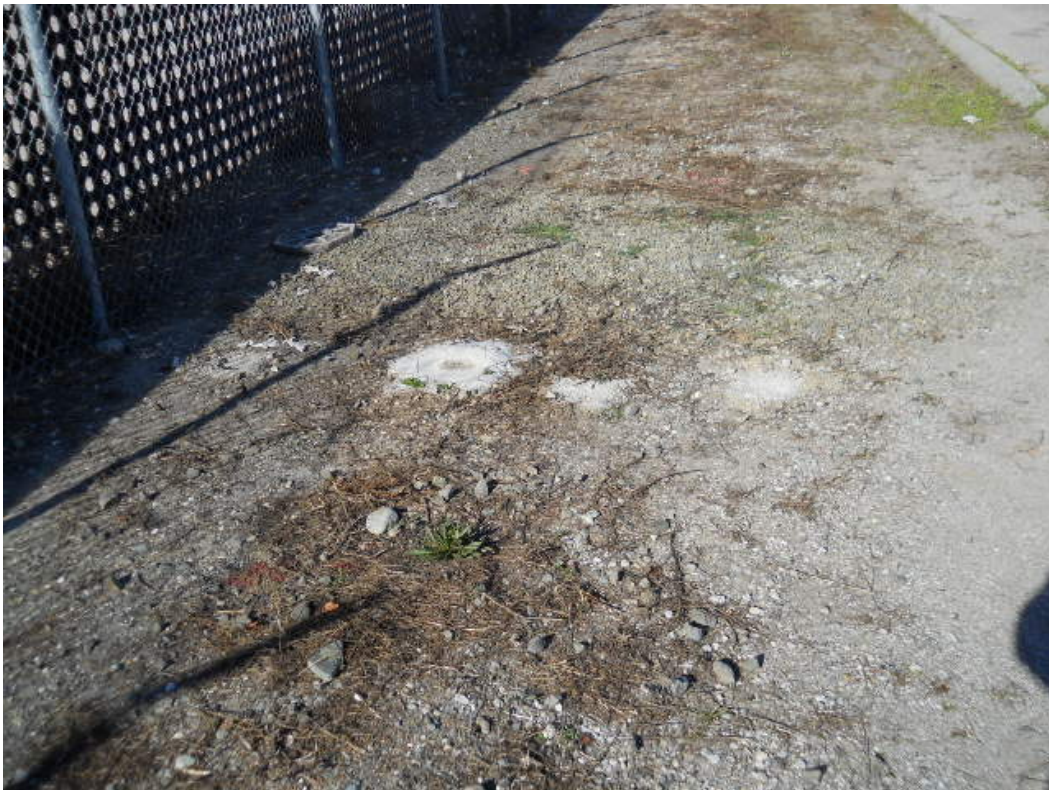
Photograph D-16. HydroPunch locations on both sides of the pipeline trench
