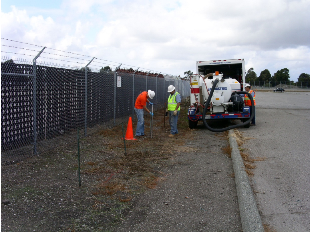
Photograph D-15. Sampling along pipeline
