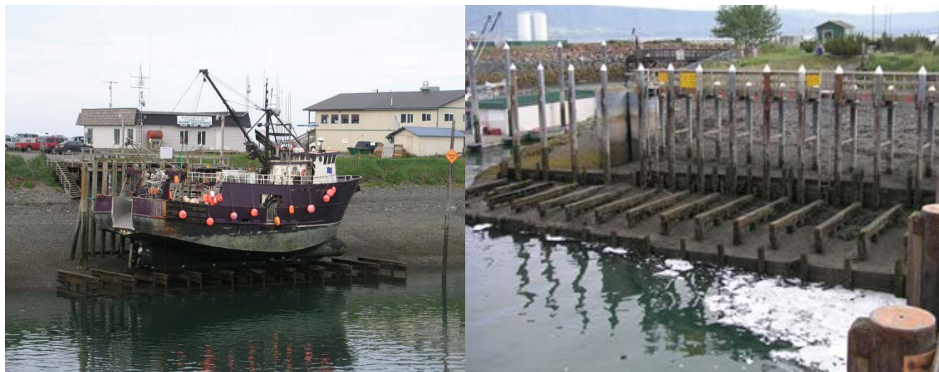
Figure 6. Grids used for boat hull cleaning and maintenance operations in Homer Harbor.
