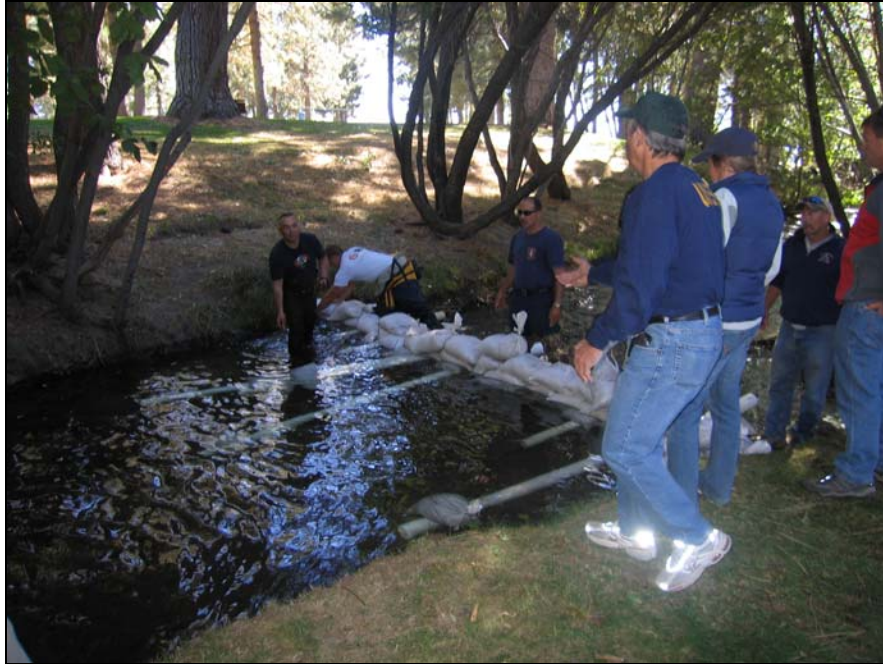
Site: Third/Rosewood Creek at Ski Beach (Photo taken from at west end of Ski Beach Park, showing an underflow dam)
