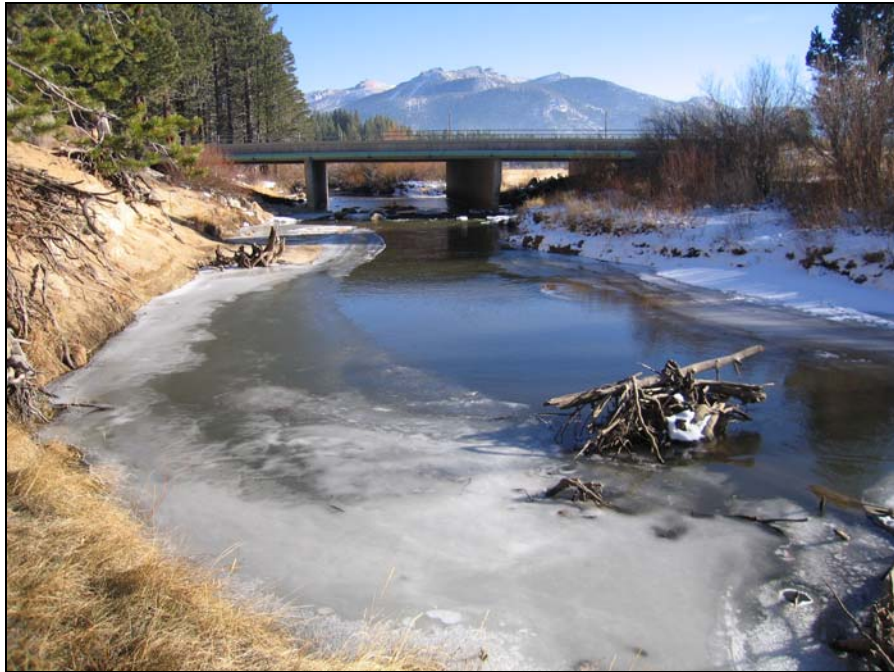
Site: Upper Truckee River Site #12 – Highway 50 Amusement Park (Photo taken from the east bank, looking upstream at the bridge)
