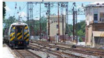
Harrisburg Line Interlocking Improvements
