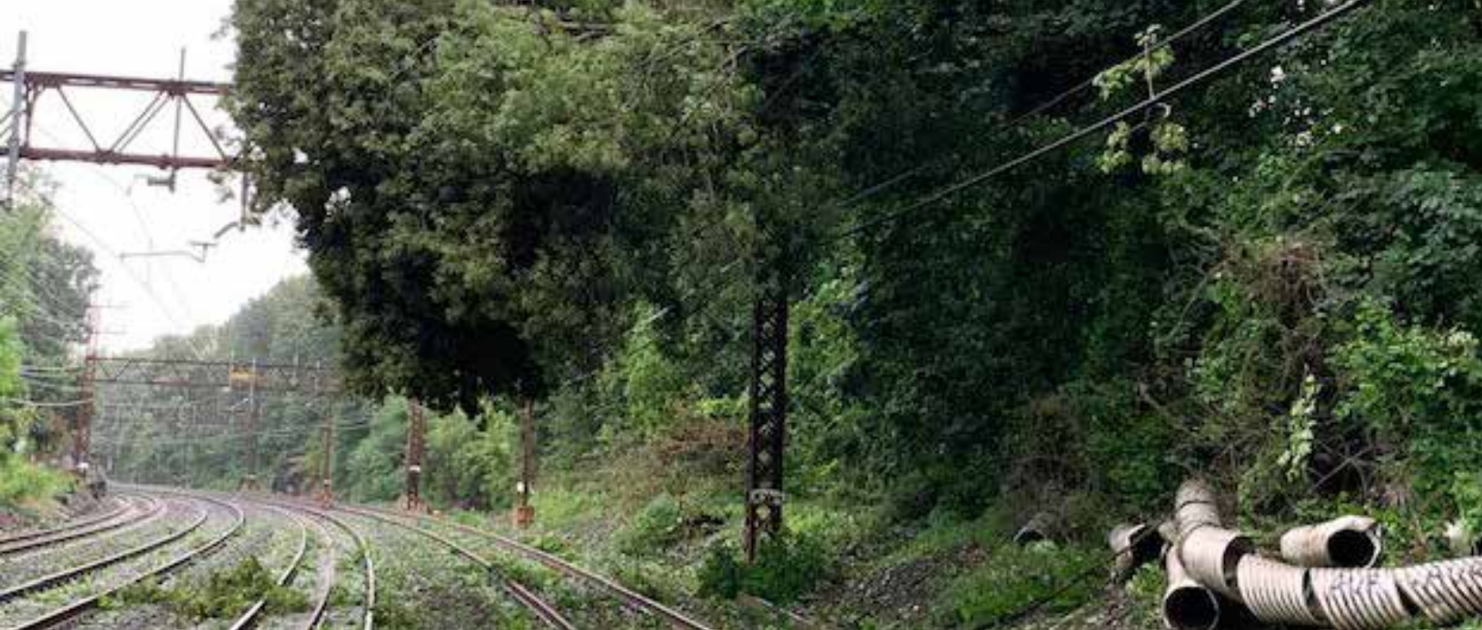
Above: MTA Metro-North Railroad crews worked for several days in August 2020 to remove trees that fell across the New Haven Line tracks because of rain and high winds from Hurricane Isaias. The hurricane disrupted NEC service across three states.
