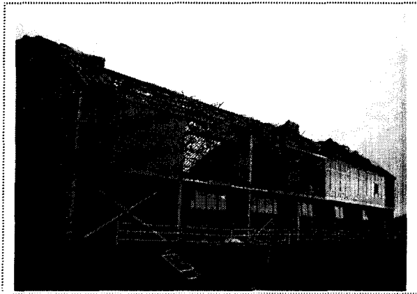
Fig.7 Example of Building Damaged by Typhoon Bart (Sep. 1999) The maximum instantaneous wind speed in Japan was recorded 83.9m/s.
