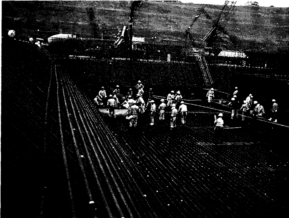
Fig. 4 First Concrete Casting for Shaking Table Foundation (June 20, 200)
