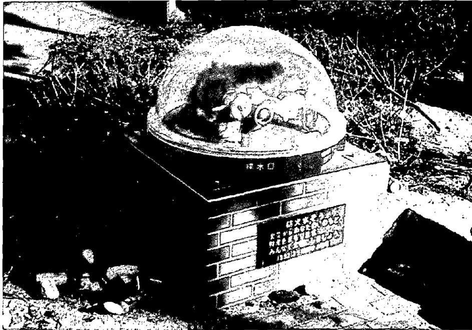
Photo 1 Cistern for water for fire protection in Kobe.
