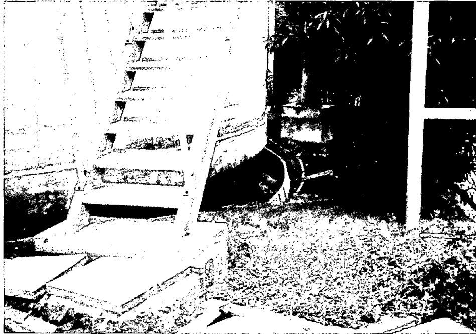
Photo 37 Differential settlement between pipe and non-pile supported structures damaged piping throughout the plant.
