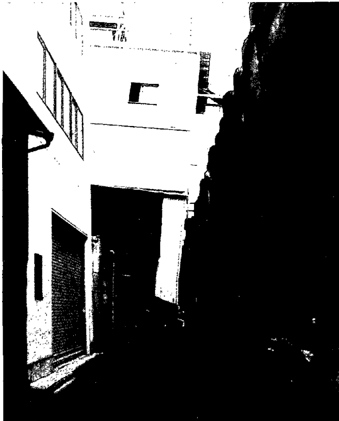
Figure 6.2.23 Road blocked by three story building.
