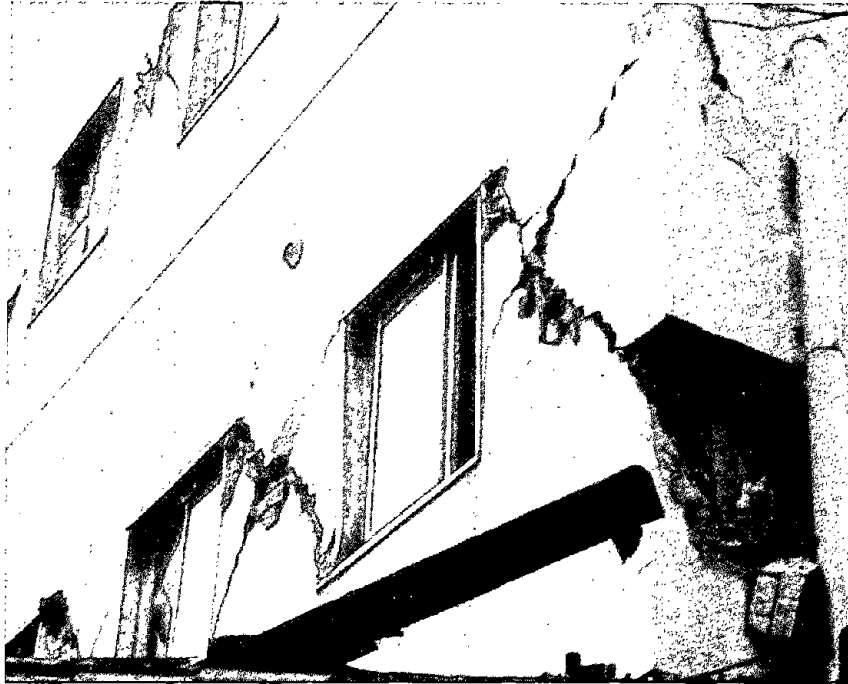
Figure 3.4.4 Diagonal tension cracks - apartment building in Nishinomiya area.
