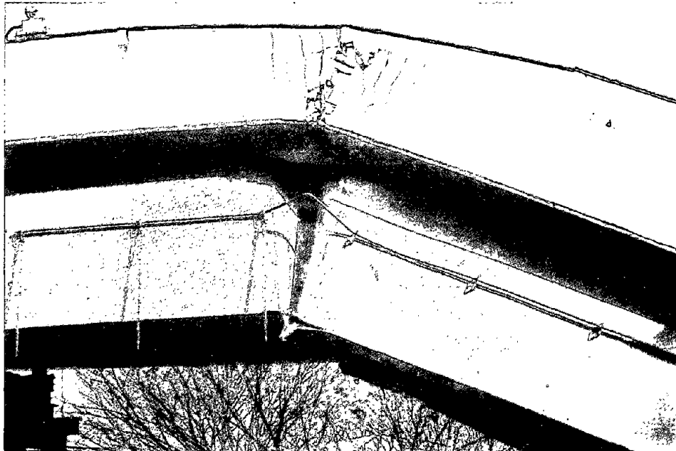
Figure 4.2.29 Girder web failure due to unseating of the Southeast Ramp at Minatogawa Interchange.
