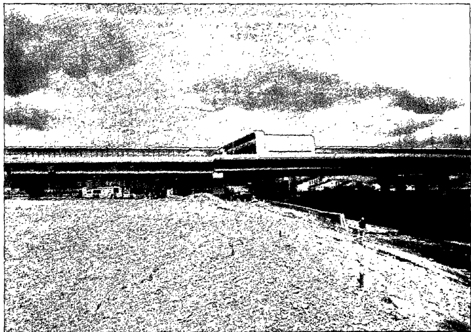
Figure 4.2.42 Distant view of the Shukugawa Bridge showing lateral deformation of the foundation soils and spreading to the right (to the center of the channel).
