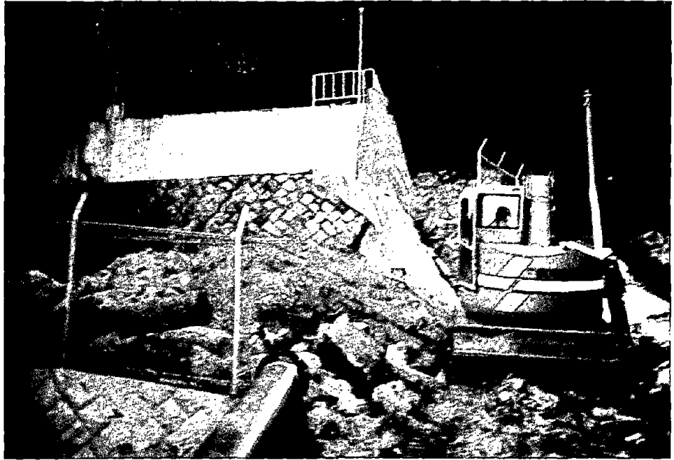
Photo 13 Broken lines to/from backwash tank at the Motoyama Water Purification Plant.
