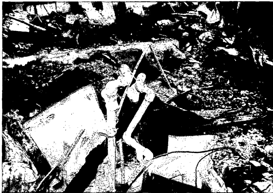
Figure 6.2.4 Broken gas meter connection.
