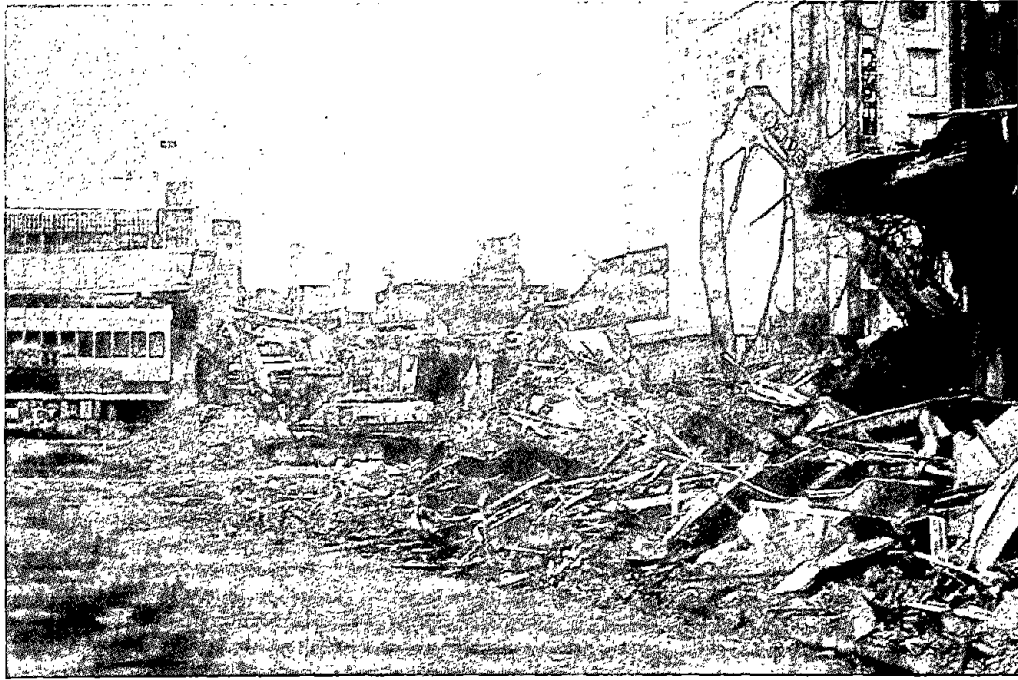
Figure 4.3.11 Collapsed Shin - Itami Station.
