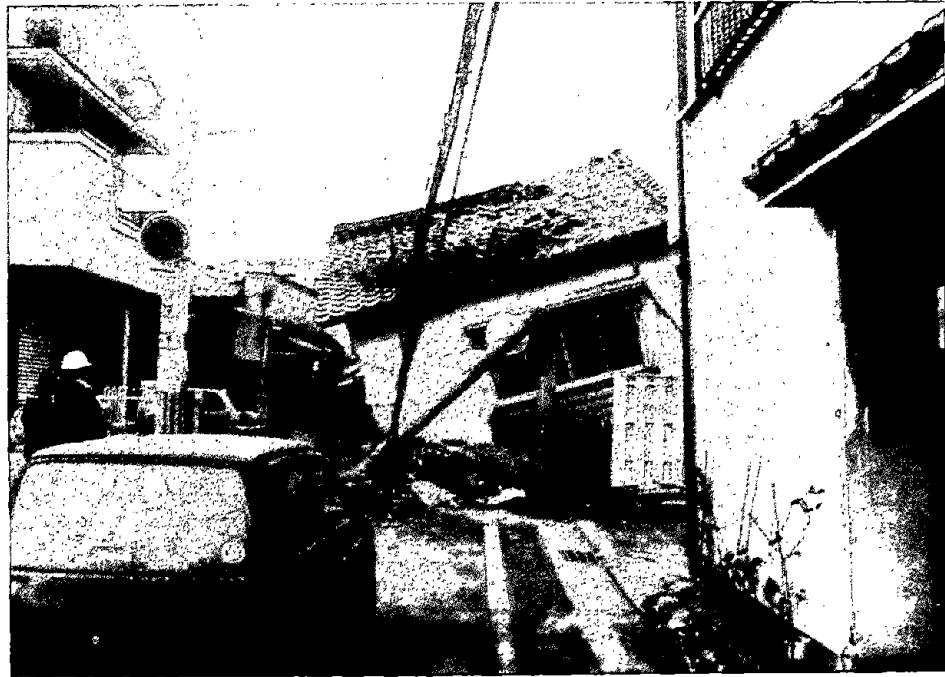
Figure 6.2.7 Example of electric power lines connected to a damaged house.
