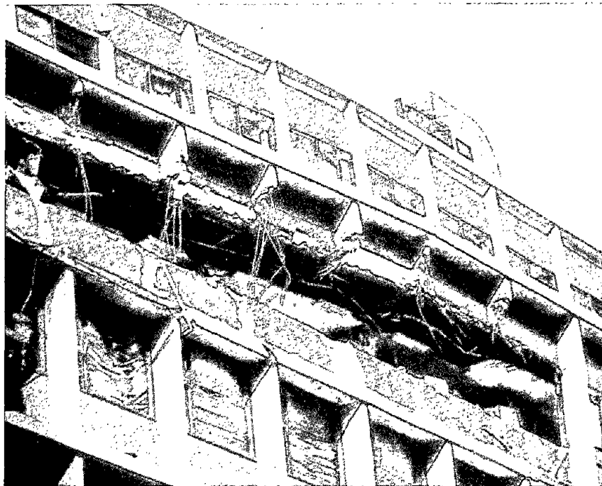
Figure 3.4.22 Upper story collapse - Downtown Kobe.
