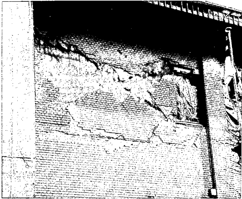
Figure 3.4.2 Damage to shear walls - Kobe Central Post Office.
