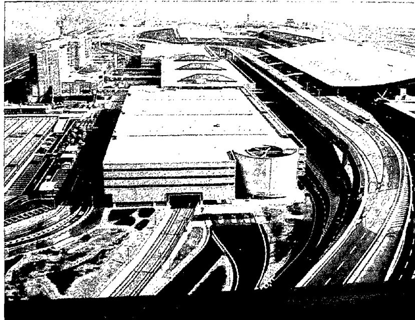
Figure 4.4.1 Overview of airport looking east from control tower.
