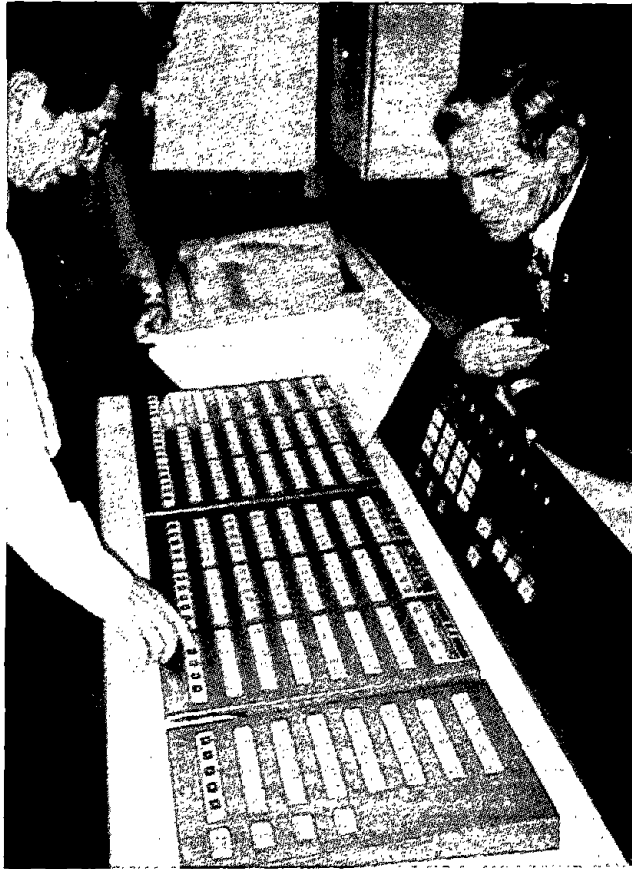
Photo 6 Control Panel for earthquake valves to provide flexibility to control automatically or by operations staff in Okuhirano Control Center.
