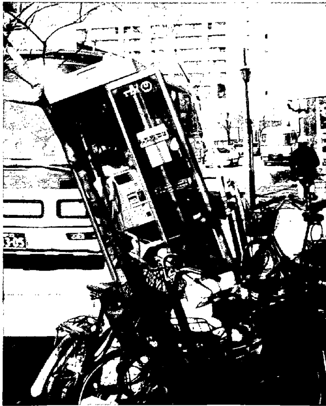
Figure 5.5.12 Soil instability damaged telephone booths.
