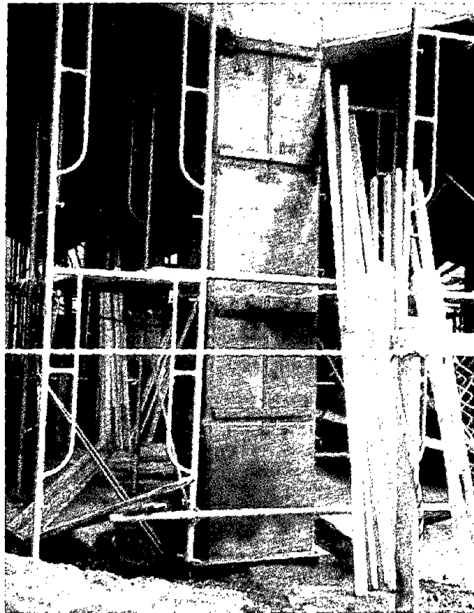
Figure 4.3.8 Jacketed column - JR Main Line.
