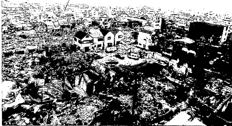
Figure 6.2.3 View of post earthquake fire damage in Nada Ward, Kobe (Site No. 8).
