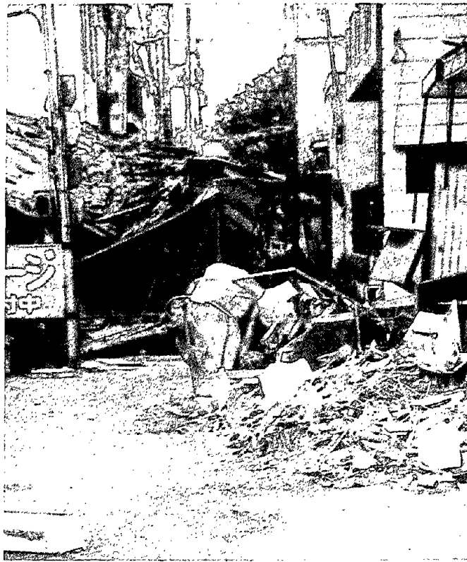
Figure 6.225 Road blocked by collapsed structure.
