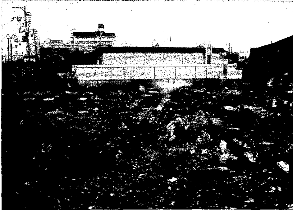
Figure 6.2.17 Electric Power Sub-Station.
