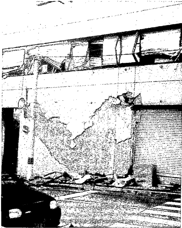
Figure 3.4.17 Second story collapse - Miyagi Hospital.
