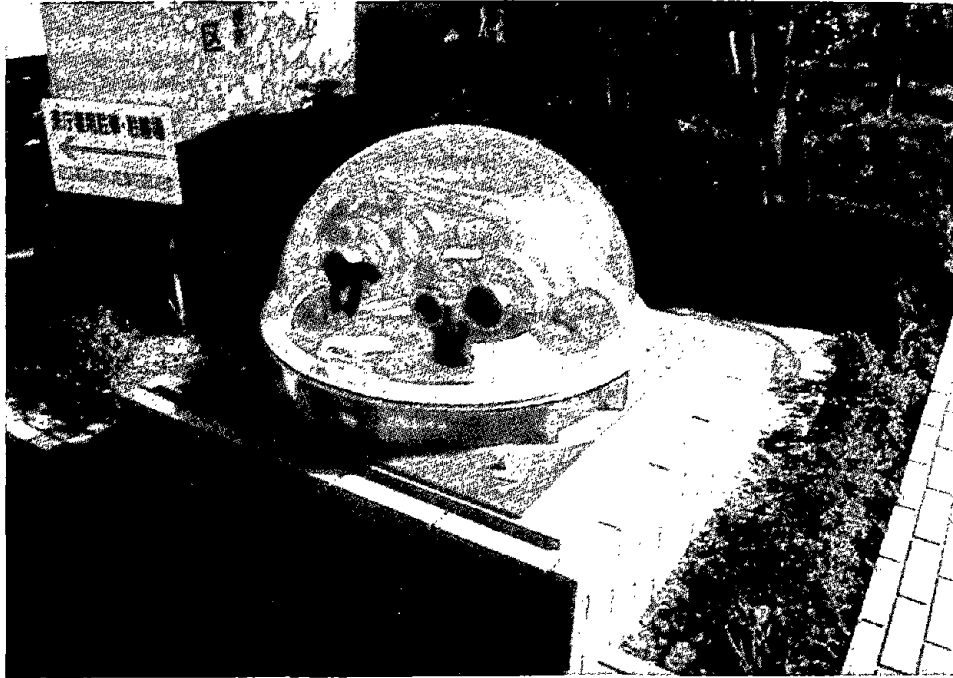
Figure 6.2.21 Seismically reinforced fire fighting water cistern.
