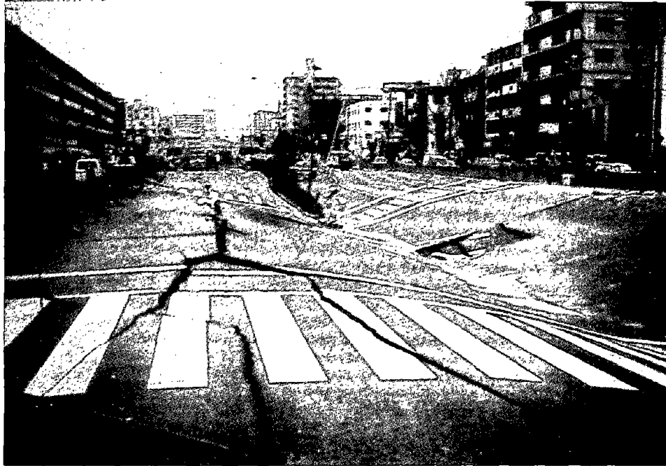
Figure 4.3.21 Subsidence of street surface over the collapsed Daikai Station.
