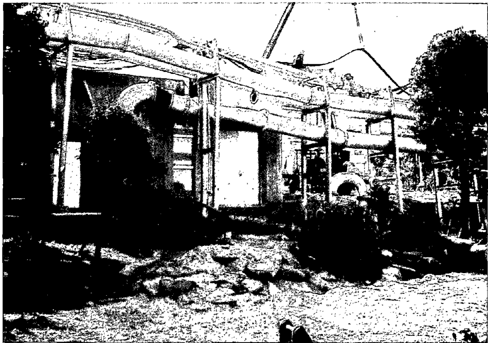
Photo 38 Filter building support pipes failed allowing the building to move and settle differentially.
