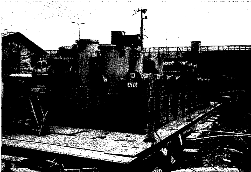
Figure 5.4.65 A 77 kV and 6.6 kV gas insulate distribution substation.
