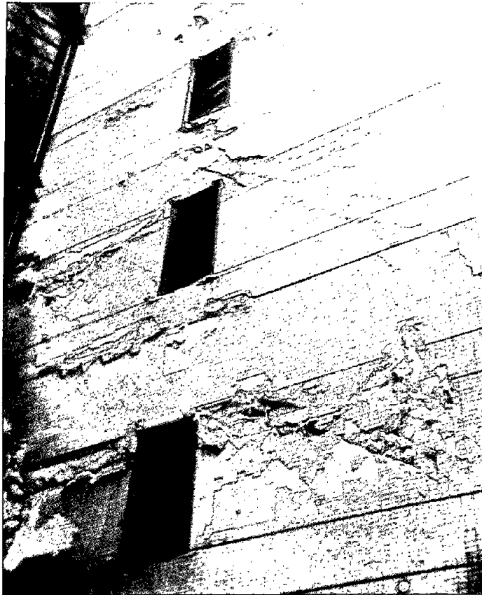
Figure 3.4.3 Damage to shear walls - office building in downtown Kobe.
