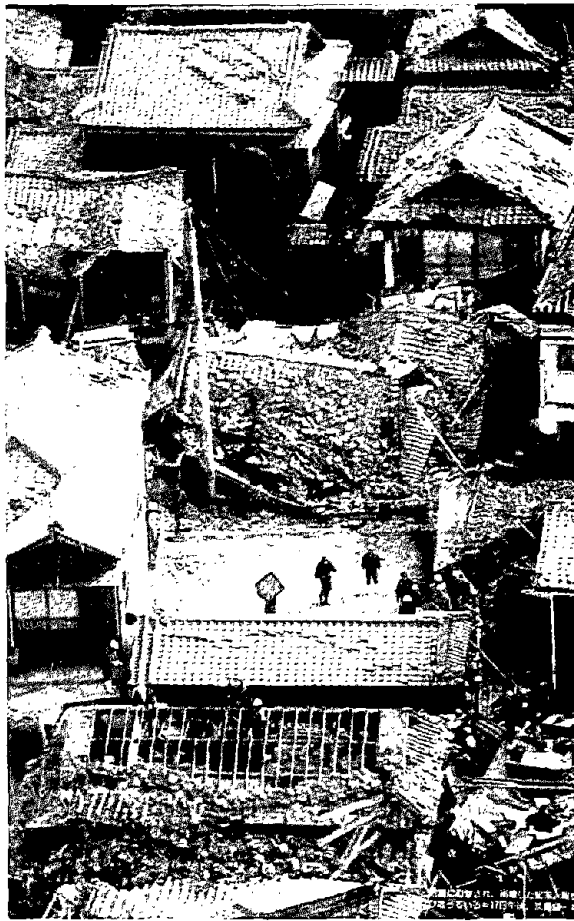
Figure 3.3.7 Collapse of some heavy tiled roof houses - Shinkabe construction.
