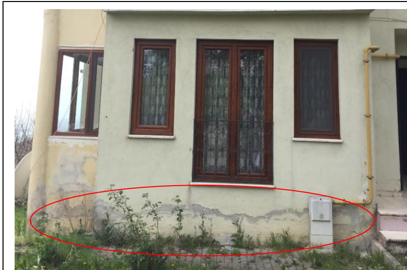
Fig.8 Type-1.1 efflorescence(northeast)
