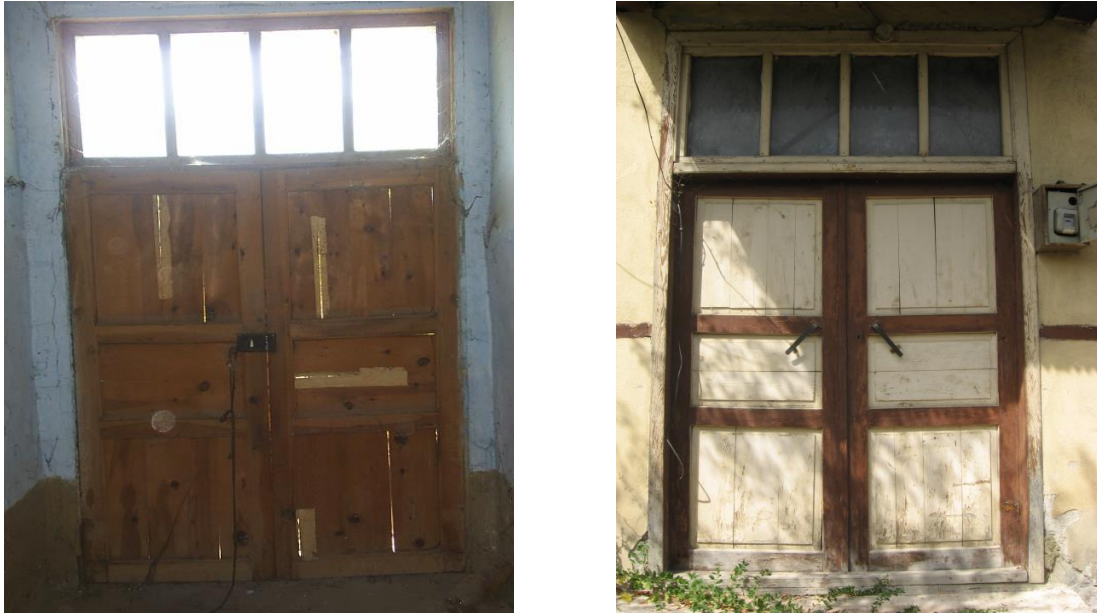
Figure 17. Ibrahim Pilavcı House of entrance door from inside and outside views.
