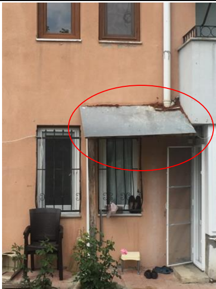
Fig.24. Type-2.2 Eaves attached to the facade (southeast)
