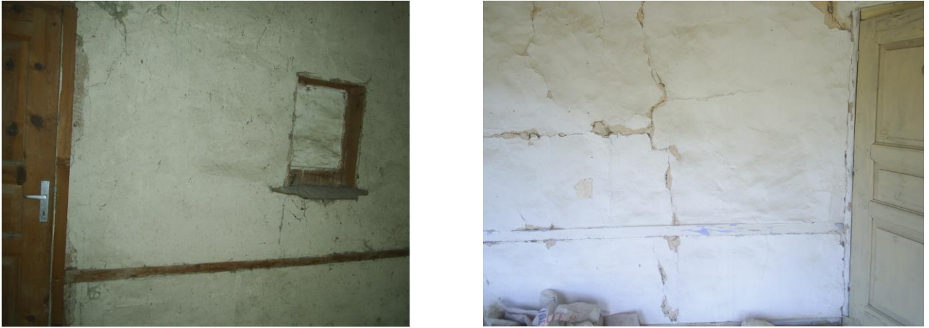
Figure 19. Ibrahim Pilavcı House of wall views.
