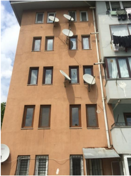
Fig. 22. Type-2.2 facade view (southeast)
