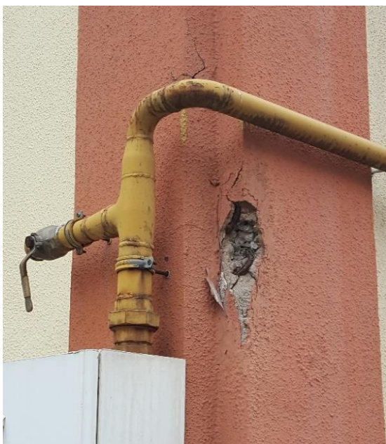
Photo 7. Damage due to building renovation.
