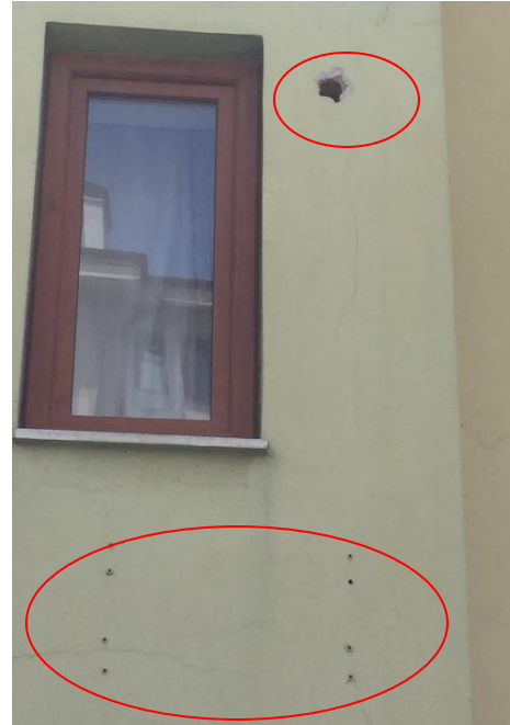
Fig.23.Type-1.2 anchor materials and drilled holes
