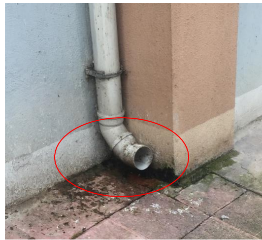
Fig. 27. Type-2.2 rain downpipe (northwest)
