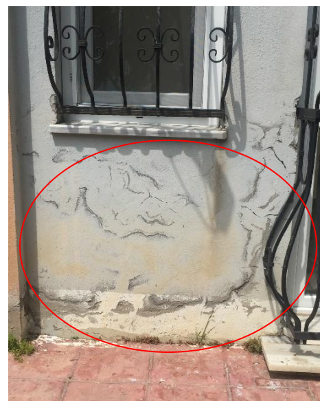
Fig.11 Type-2.3 efflorescence(northwest)
