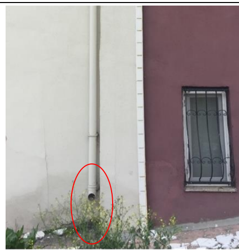
Fig.29. Type-2.1 rain downspout (northeast)
