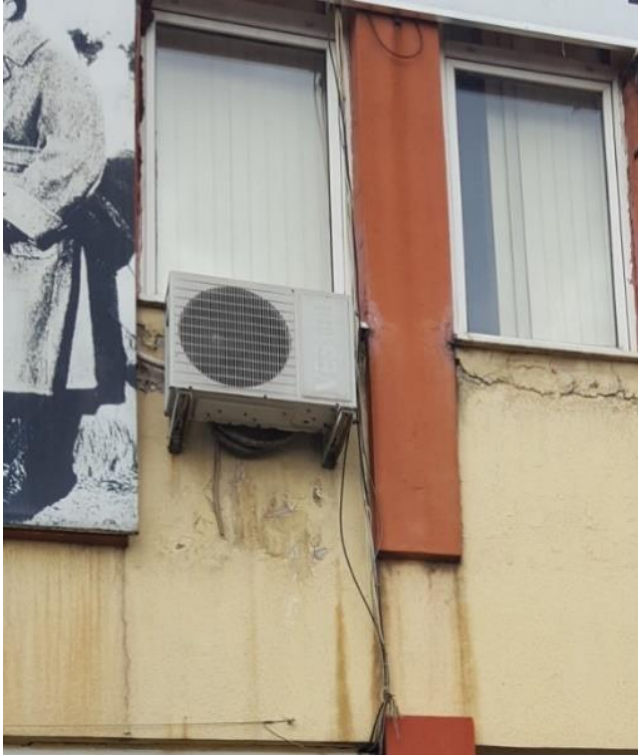
Photo 6. Incorrectly applied air conditioning application.
