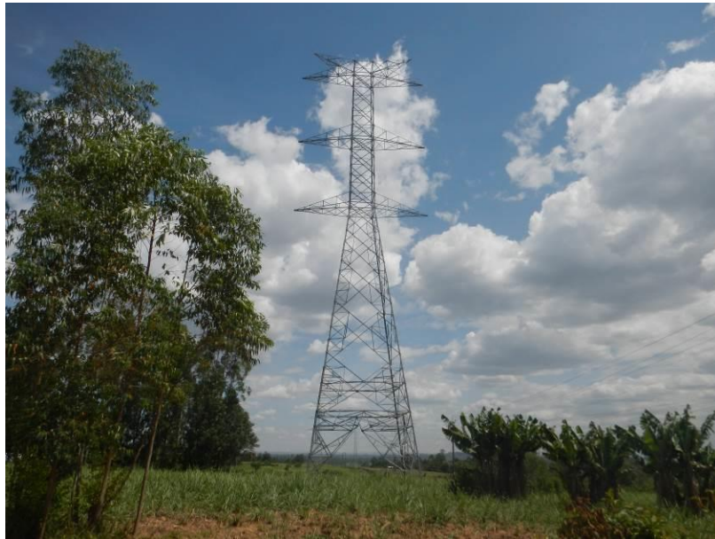
Plate 22: KETRACO transmission line pylons in the project area
