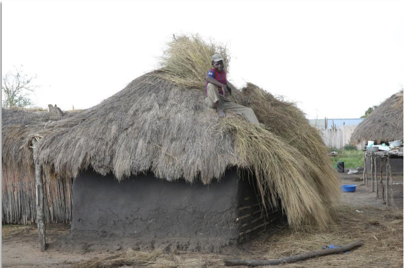
Figure 8: Traditionally built house in process of being thatched
