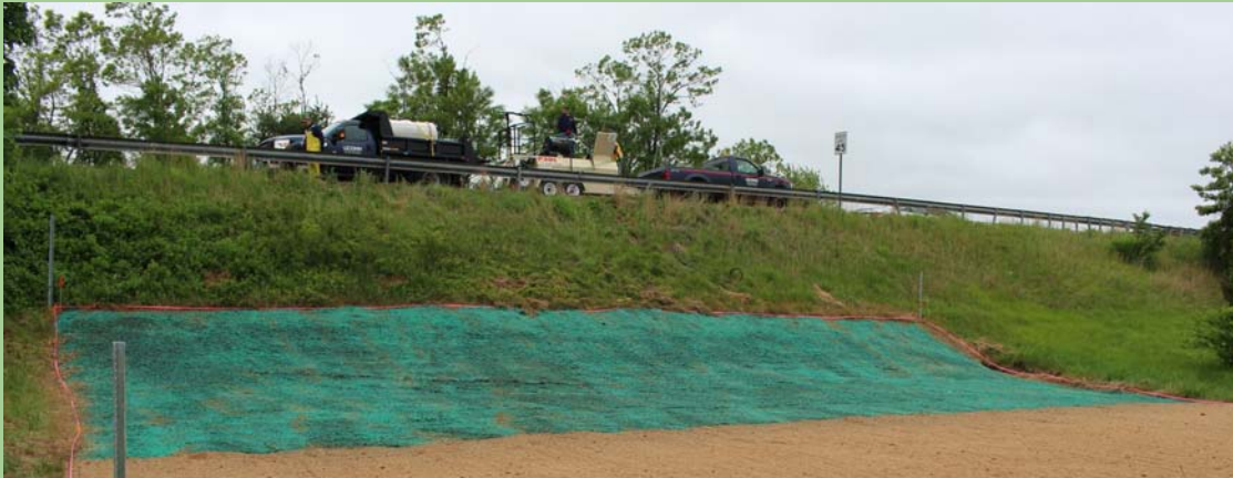
Figure 3.6 Hydroseeded slope along US Route 6.
