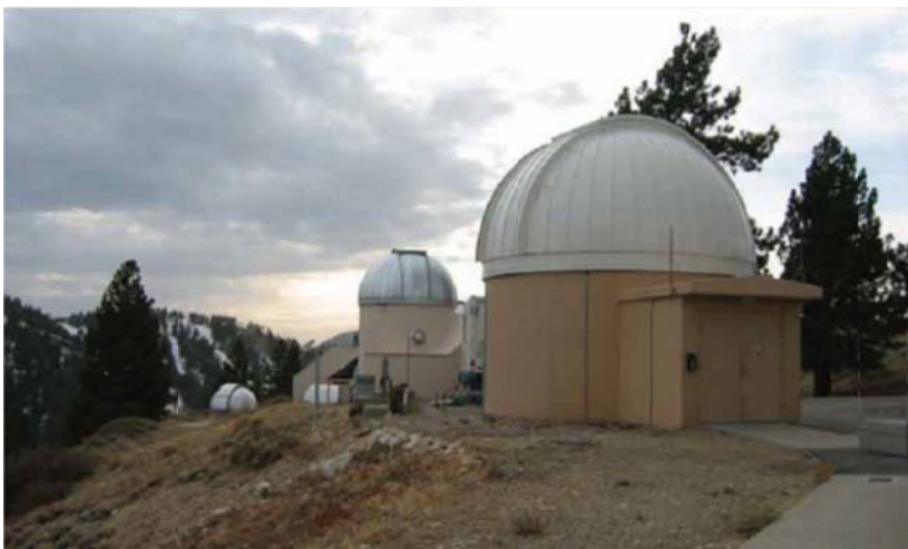
Figure 3-16. Building TM-23 atop Table Mountain Ridgeline
