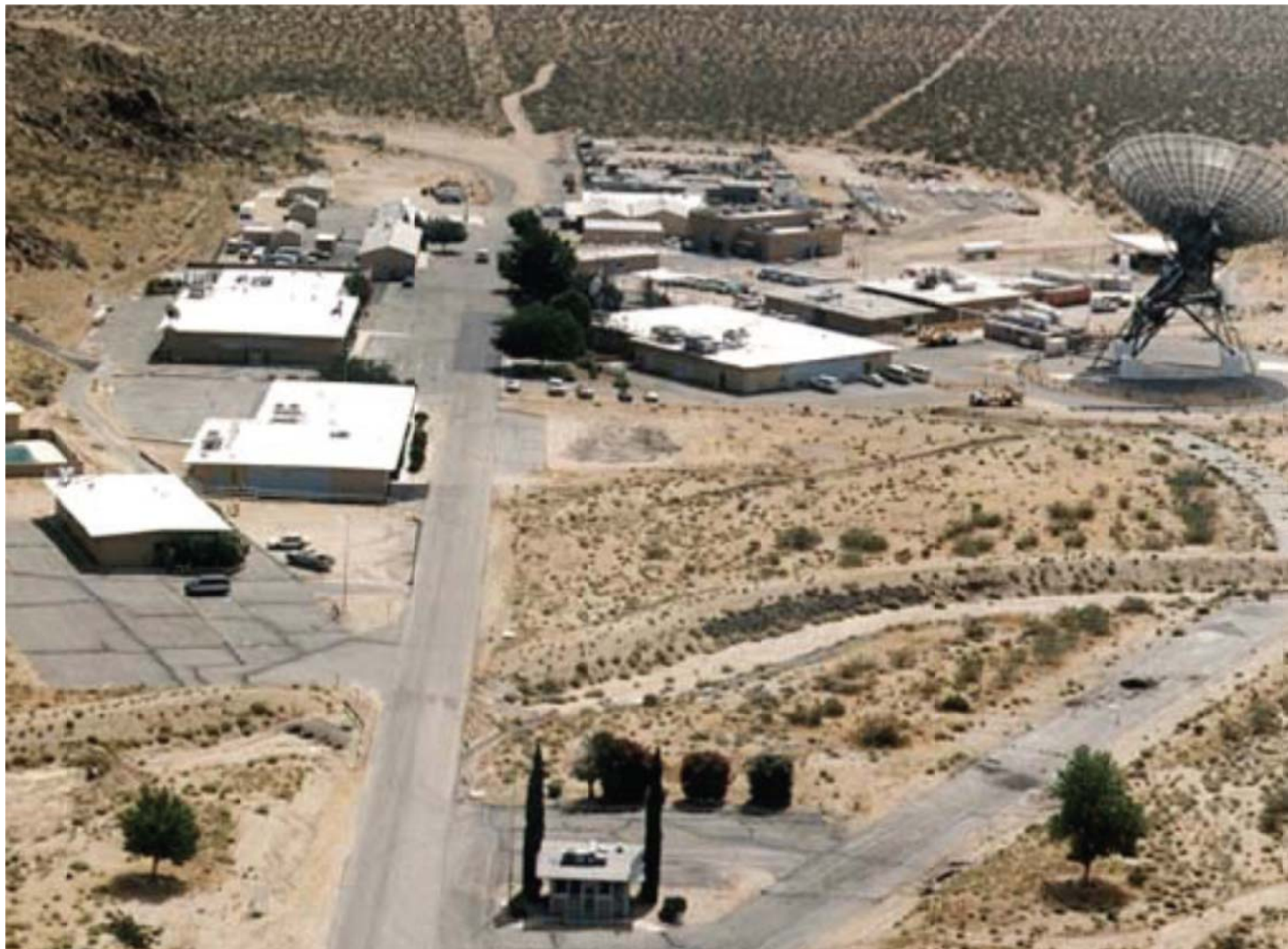
Figure 3-25. Photo of Echo Site, GDSCC
