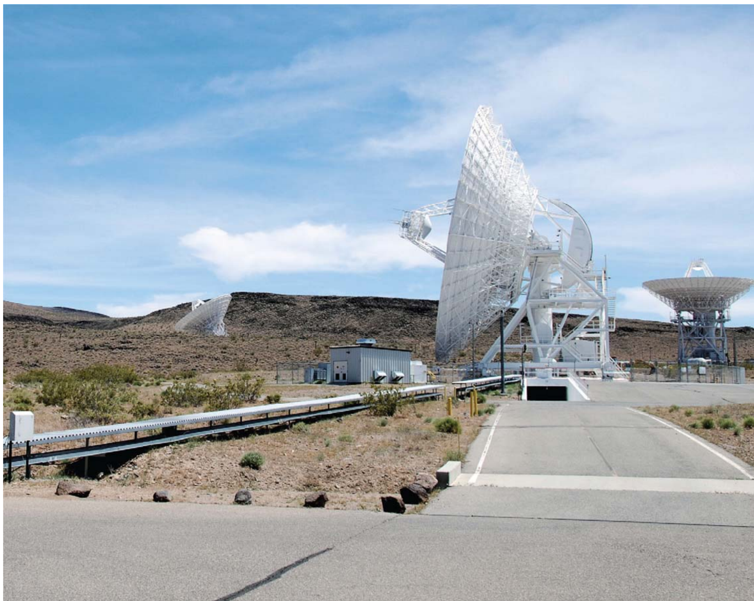
5289 Figure 3-30. DSS-25, 34-m (111.5-foot) BWG Antenna at Apollo Site, GDSCC
