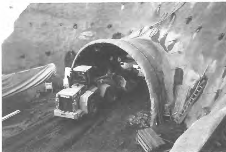
Nordre portal, toppstoll Photo from northern portal, top heading
