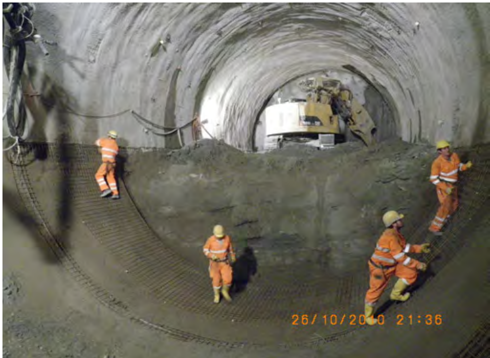
Figure 3 Invert works at contract lot KAT 1
