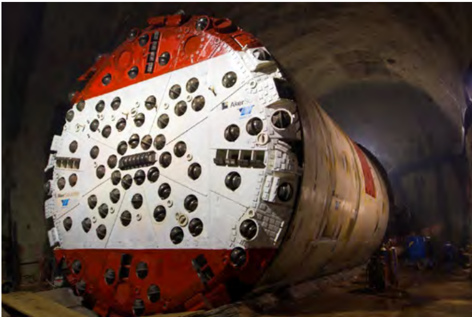
Figure 4 TBM "south" right after installation in lot KAT 2
