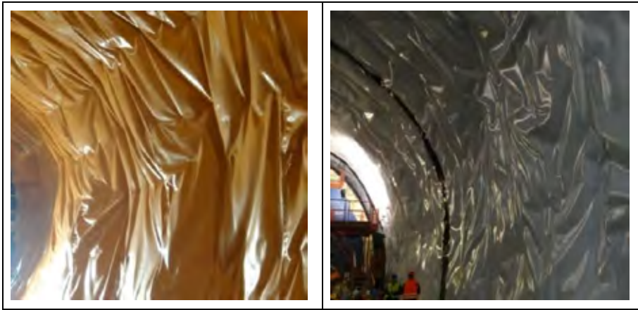
Figure 15 A degree of 3D adjustment is evident in these NATM-style membrane photographs, allowing the concrete to increase to at least 1 m thickness, instead of the 35 or 40 cm as typically designed in inevitably unrealistically uniform numerical models.
