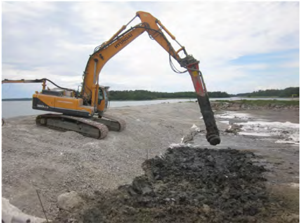
Figure 2. Mass stabilisation in the Port of Yara in Uusikaupunki in 2014
