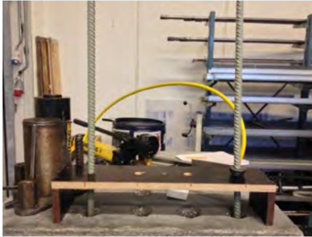
Figure 3 – Frame is used to keep the bolts from dropping into the holes and keep the vertical while the grout hardens.
