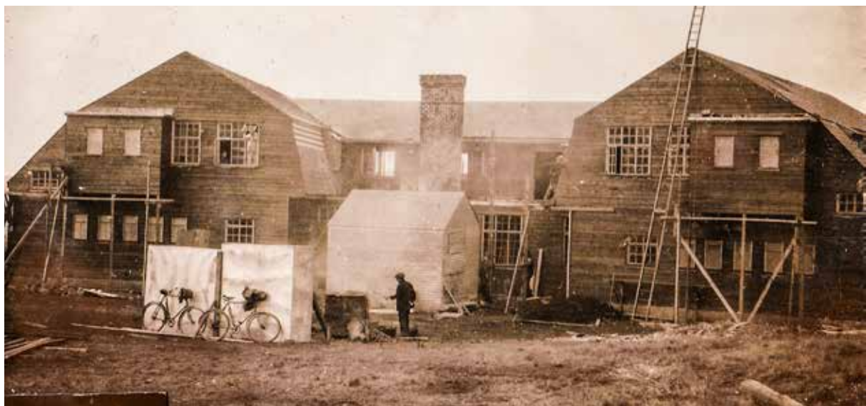
The Holiday Fellowship under construction, 1930s.
