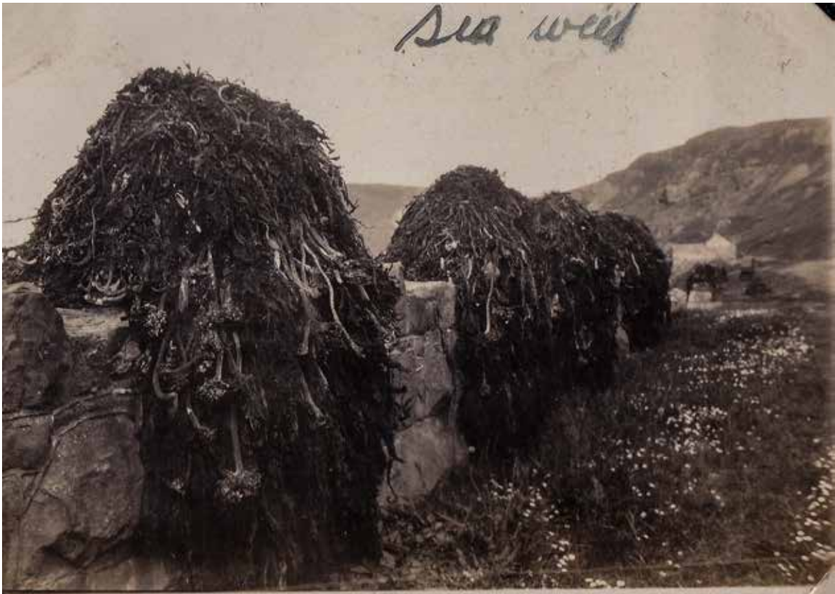
A more recent version, c.1940. This is the wall just before the car park at the old Coalyard (in the background).
