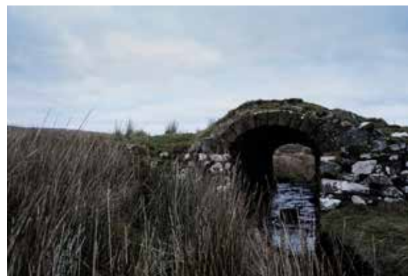
Bridge over the Drove Road at Inispollan (Cushendun), December 2018.
