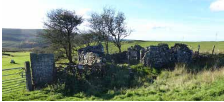
Paddy Roe's, an old shepherd's house near the Hungry House in Ballyvenagh.
