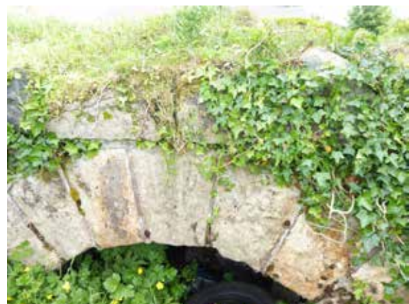
Mill race tunnel below the road.
