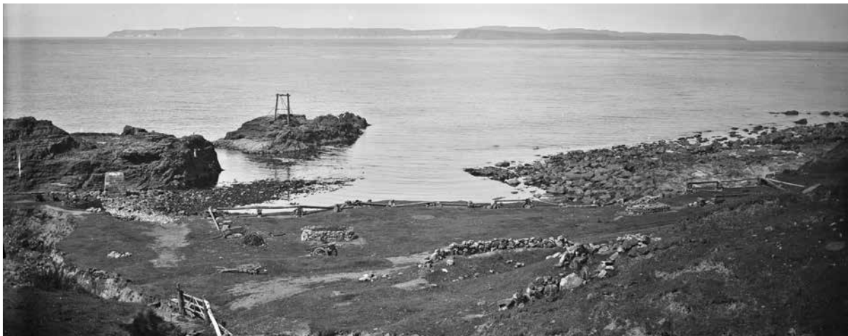
Carrickmore c.1900, two stone kelp pits can be seen in the Hearths. Courtesy of the National Library of Ireland.
