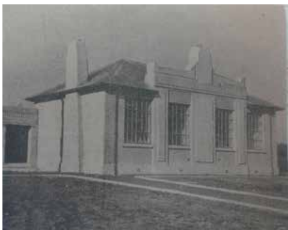
The newly opened Barnish Primary School, 1935.
