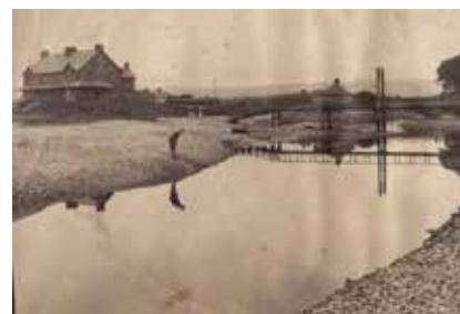
The old border crossing, built by the Dallat brothers of the town c.1905.
