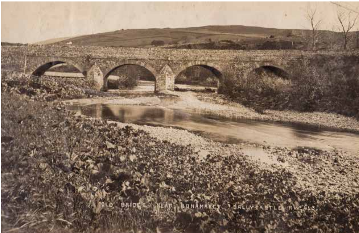
The Drumahaman bridge from the Bonamargy side c.1900.
