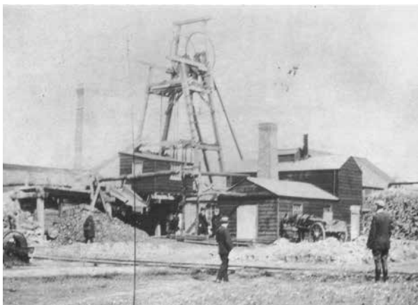
Tracks in the foreground for the carts.
