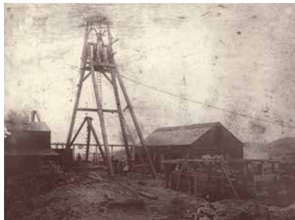
Pithead, from Danny McGill's Moyle Memories. The operator can be seen at the top of the winding gantry, which controlled the carts ascending and descending the mine shaft.
