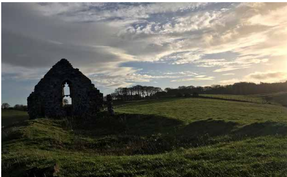
The chancel gable 2018. The remaining gable is thought to be a reinforcement of the original building, as the ground is sandy and full of springs.
