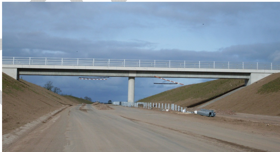
Figure 4-2 Typical Two Span Open Aspect Structure
