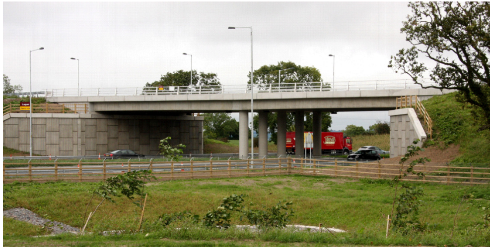
Figure 4-4 Two Span Closed Aspect Overbridge Structure
