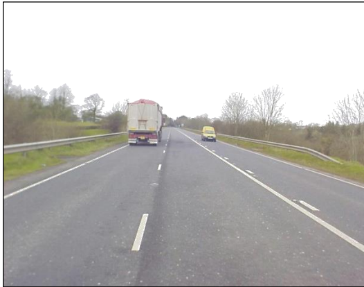
Figure 2-33: Northbound Climbing Lane north of Ballygawley Roundabout
