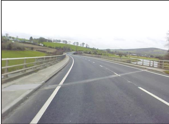
Figure 2-19: River Strule Northern Crossing, Newtownstewart Bypass
