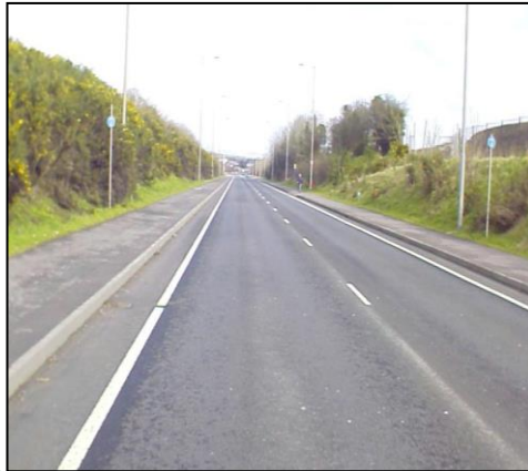
Figure 2-7: Combined footway and cycleway on either side of the A5 at Strabane Bypass
