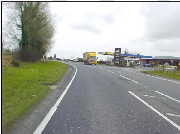
Figure 2-20: Existing A5 with Central Hatching, Mountjoy
