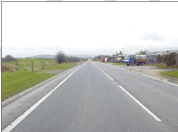
Figure 2-18: Existing A5 North of Newtownstewart
