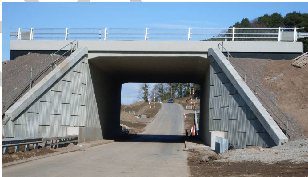
Figure 4-5 Closed Aspect Underbridge
