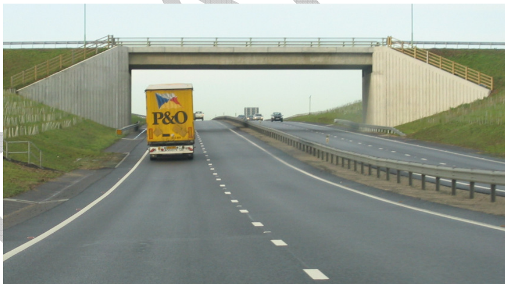
Figure 4-3 Single Span Closed Aspect Overbridge Structure
