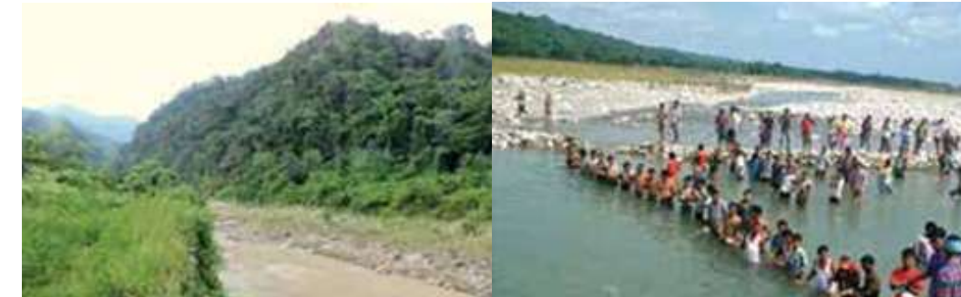
A river during its peak flood season Construction of dong bundhs before dry spell
