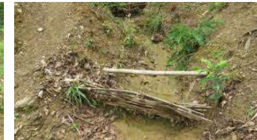
Water channel with bamboo check dam made to control soil erosion
