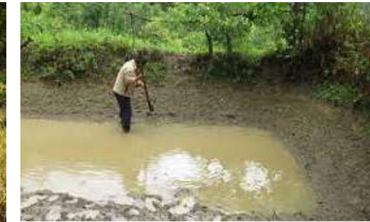
Using a pole tied to a gunny bag, a farmer rams and compresses the side wall of a pond
