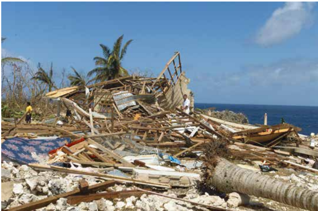
FIGURE 18. Damage caused by Cyclone Heta.
