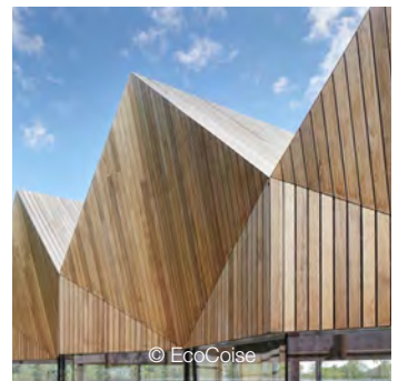
Picture 7: Alfriston School, Buckinghamshire (UK). The outside paneling including the roof is made with thermally modified wood of the species Fraké - also known as Limba.
