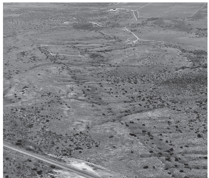
FIGURE 2.2. Aerial view of Pratt dike, east of National Parks Highway.
