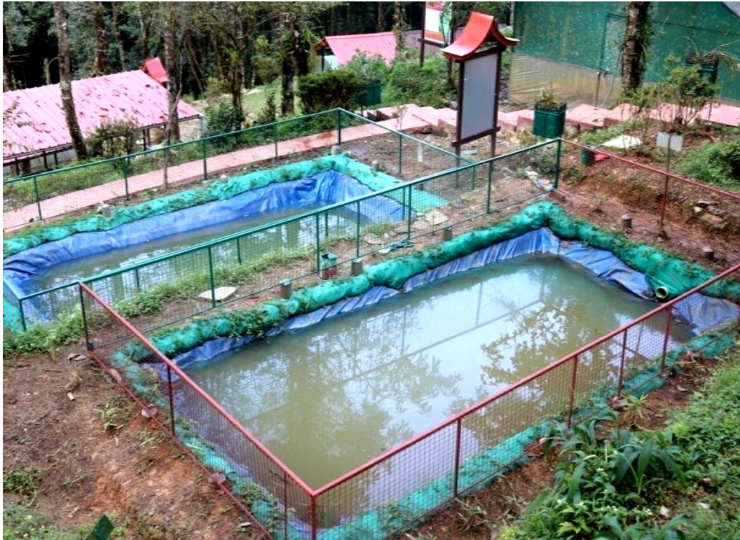
Fig: Rain water harvesting Unit at the RTC
