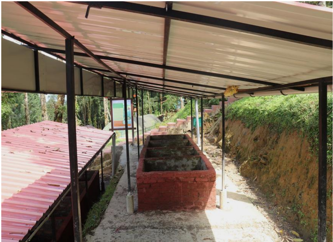
Fig: A view of vermi-composting unit at the RTC
