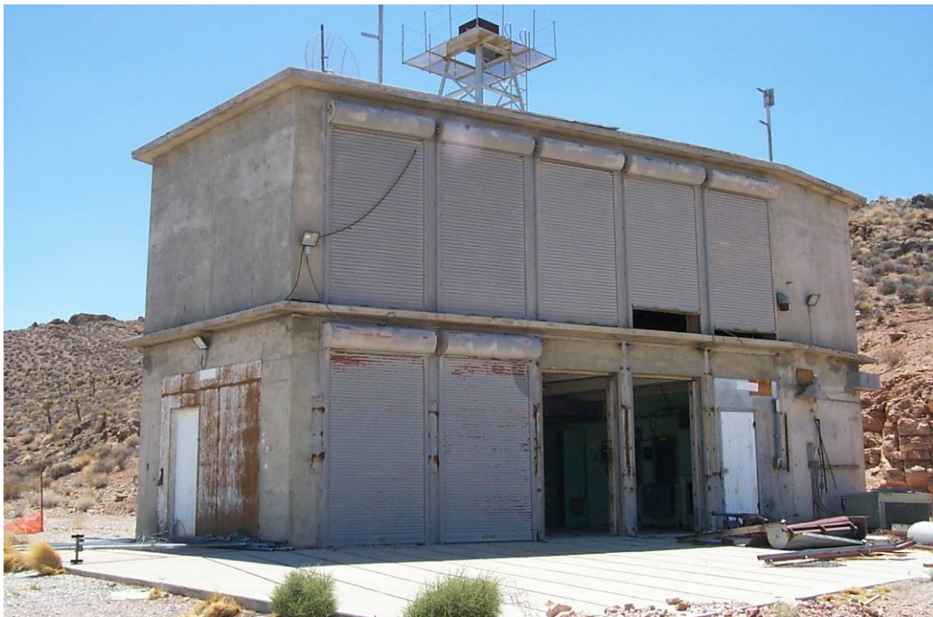
Figure A-24. Building 400, a camera station for photographing atmospheric tests, at Area 6 Control Point. Built in 1951, it was one of the first buildings constructed on the NNSS to support weapons testing activities (photo taken by DRI 2003).
