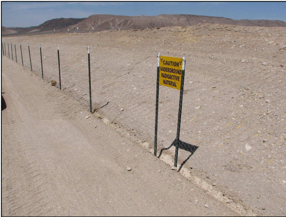
Figure 7-6. Rabbit-proof fence erected around CAU 577 Cells 19/20 to prevent herbivory. (Photo taken April 19, 2022, by D.B. Hall)
