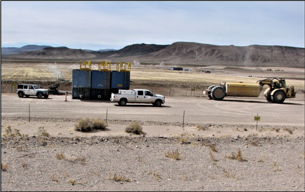
Figure 7-9. Watermaster filling water tanks at CAU 577 East Cover Cap. (Photo taken March 24, 2021, by D.B. Hall)
