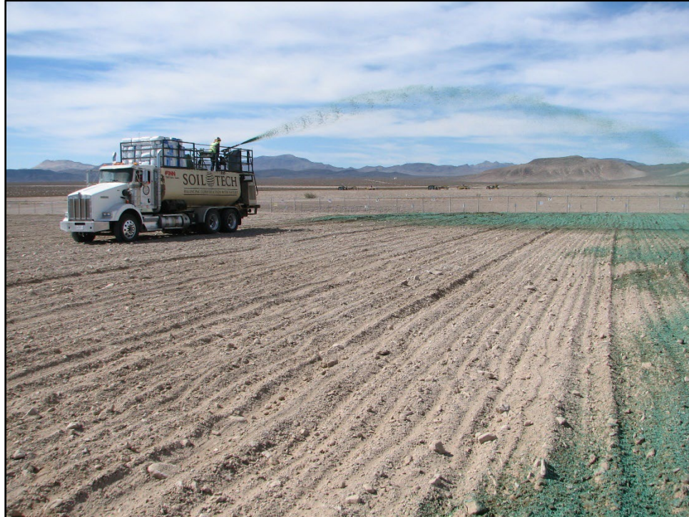
Figure 7-8. Applying hydromulch on CAU 577 Cells 19/20. (Photo taken March 8, 2022, by D.B. Hall)
