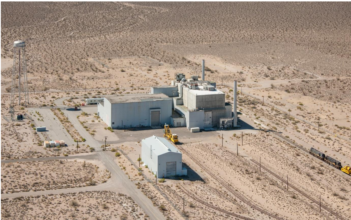
Figure A-27. The NRDS Engine Maintenance and Disassembly Building (photo taken by Remote Sensing Laboratory 2013)
