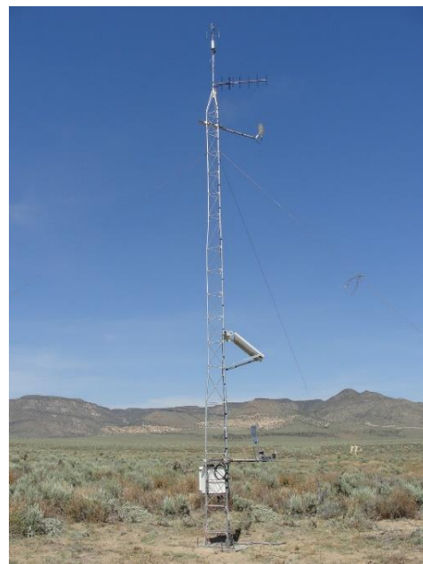
Figure A-13. Example of a typical MEDA station with a 10-meter tower
