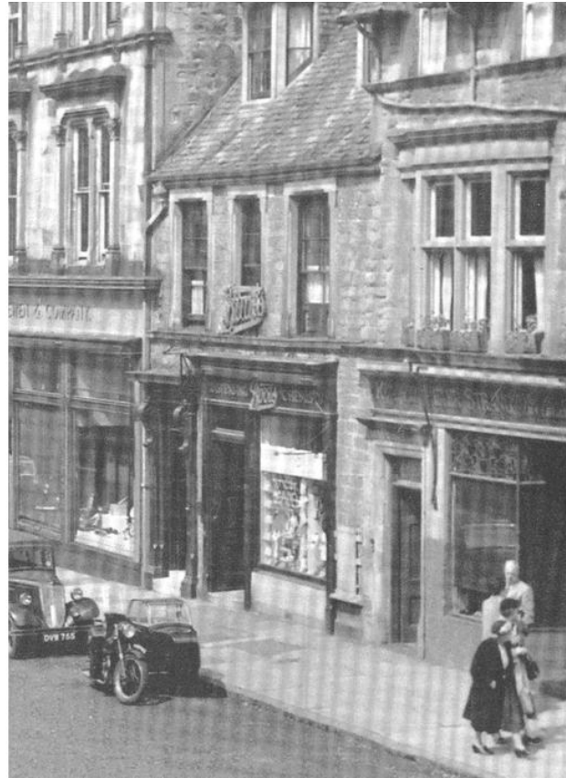
Figure 7 1950s photograph of Main Street showing the edge of the present day 'Shell Centre'. The original stonework of the first floor canted bay window is present; however, possible salts or carbonate efflorescence are visible in the stonework just above the bay window near the rainwater goods. This indicates excess water penetration beneath the wallhead dormers, most likely due to early stages of failing rainwater goods. No over painting is present at the time of this photograph (Byrom, 9).
