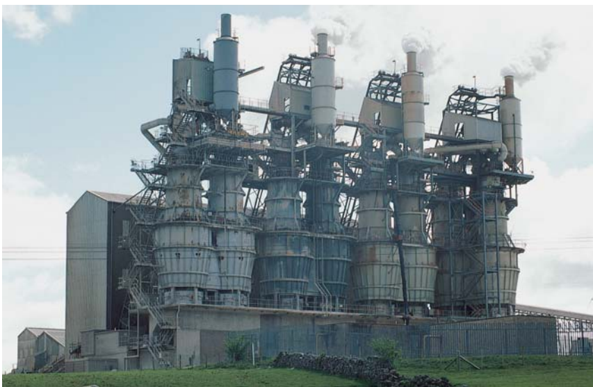
Left High purity limestone quarried at Shapfell in Cumbria feeds kilns which supply lime to a number of iron and steel plants in England and Wales.
