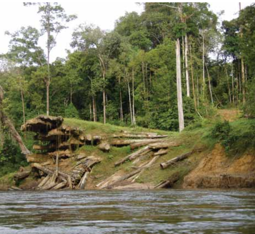
Abandoned and collapsed logging bridge. Murung River, Central Kalimantan. Photo: Stephan Wulffraat
