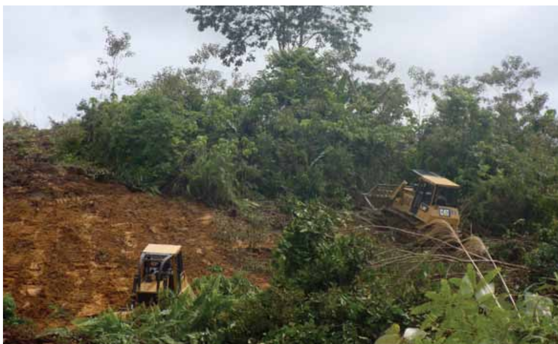
Opening land with bulldozers for establishing a new oil palm plantation. Photo: Stephan Wulffraat
