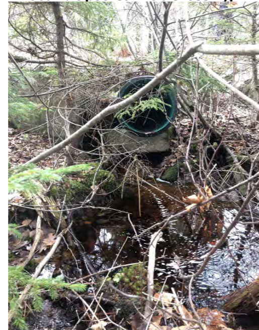
Photo 2: Downstream at Crossing, perch culvert
