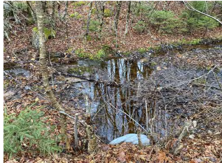
Photo 1: Culvert at crossing
