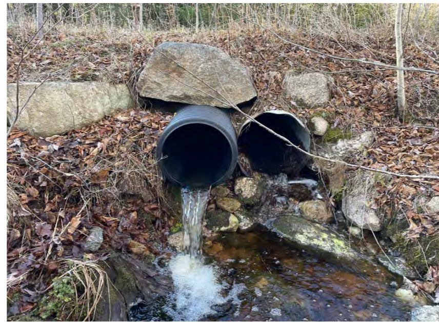
Photo 1: Perched culvert at crossing
