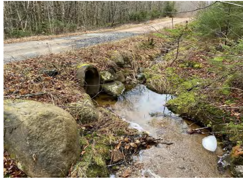
Photo 1: Culvert looking downstream at crossing.
