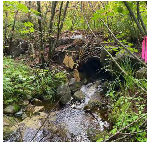
Photo 4. Evidence of alteration along WC2.
