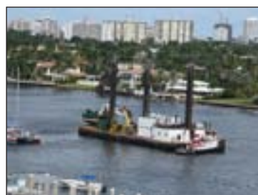
On the Cover: Cashman Dredging Company's backhoe dredge Captain A. J. Fournier works in the Atlantic Intracoastal Waterway at Fort Lauderdale, as seen by attendees at the WEDA Eastern Chapter Meeting in November. The "Captain" dredged 180,000 cubic yards of material during the project, which started in early May and was completed on December 22, from the 17th Street Causeway to Sunrise Boulevard. Steve Tobin was project manager. Photo by Marsha Cohen.
