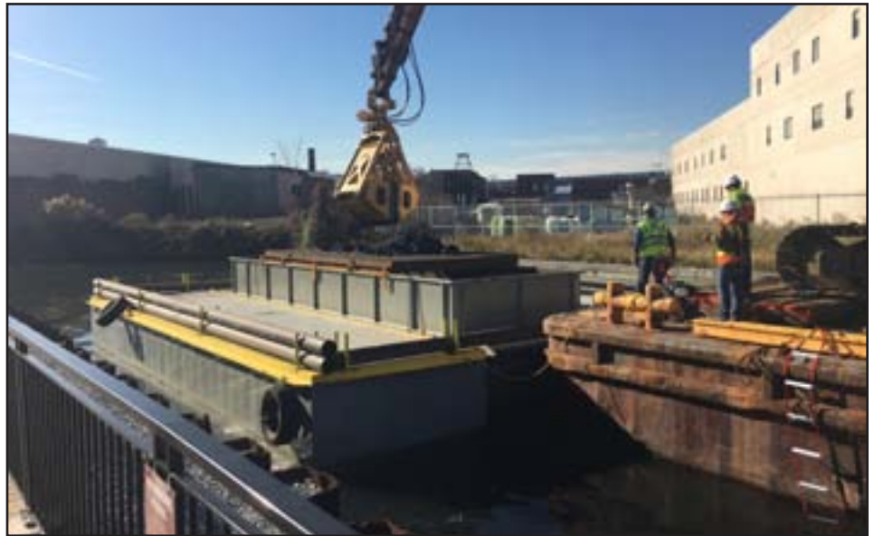
Crew members watch as a clamshell bucket deposits dredged material into a barge. This bucket is one of four that were tested in a pilot study that will enable finalization of a remedial design for the cleanup of the entire 1.8-mile-long Gowanus Canal. Photo courtesy of USEPA.
