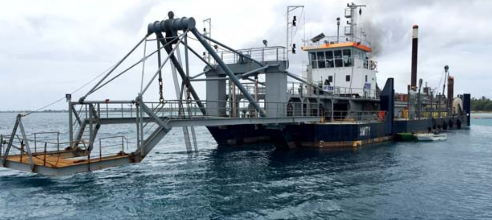
Hall Contracted used its cutter suction dredge Amity for an aid project, through the New Zealand government, at Tuvalu, a small Pacific Island country.
