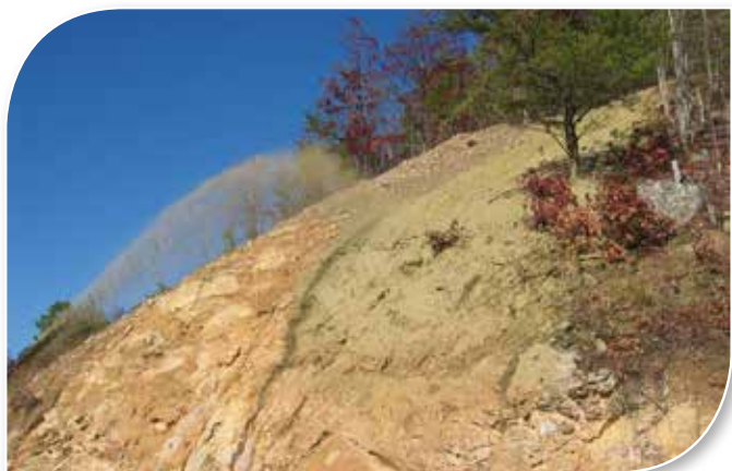
Seed mixture being hydro seeded onto the Foothills Parkway.
