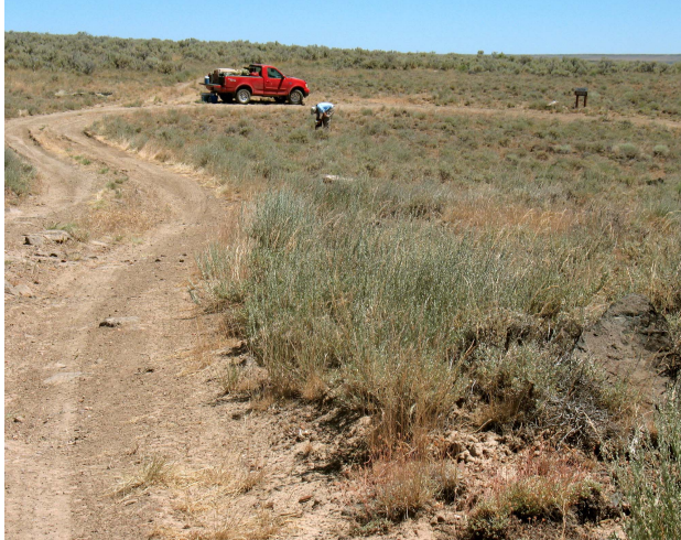
Photo 9.10. Erosion in the tire tracks of an unimproved road across the plateau in the upper Owyhee subbasin.
