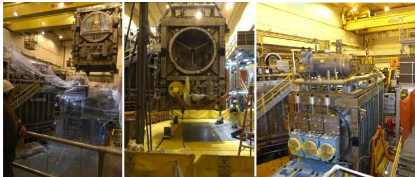
Fig. 10.15. Relocation of the 2 nd NBI beam line box. (a) The beam box lifted over the NSTX-U Test Cell. (b) The beam box being lowered into the final position in the NSTX-U Test Cell. (c) The beam box being assembled.
